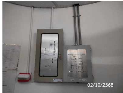
Graphic Annunciator Fire Alarm System
