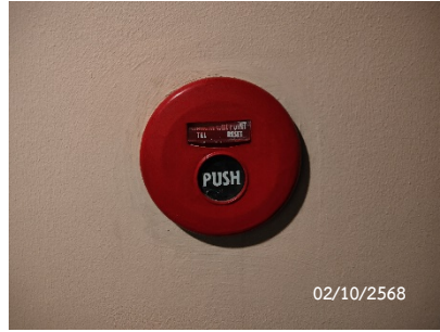
Fire Alarm Manual Station
