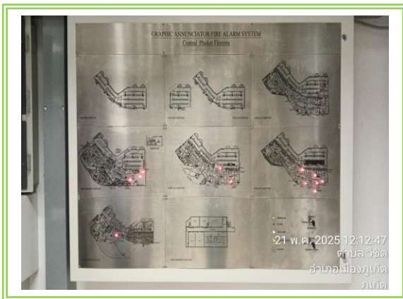
Graphic Annunciator Fire Protection System
