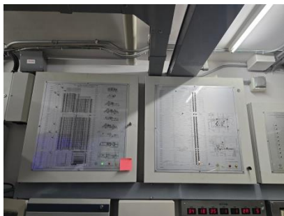
Graphic Annunciator Fire Alarm
