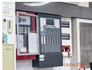
Fire Alarm Control Panel
