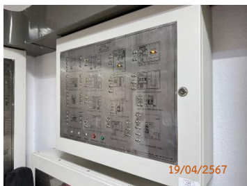
Graphic Annunciator Fire Alarm System
