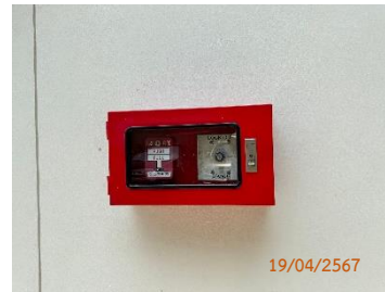
Fire Alarm Manual Station
