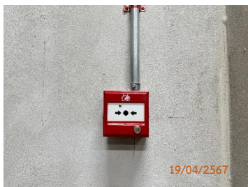
Fire Alarm Manual Station
