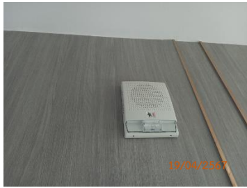
Indoor Selectable Output Speaker
