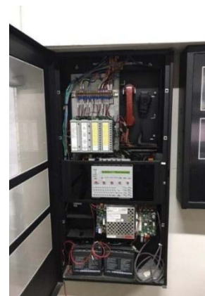
รูป2-30 Fire Alarm Control Panel (FCP)
