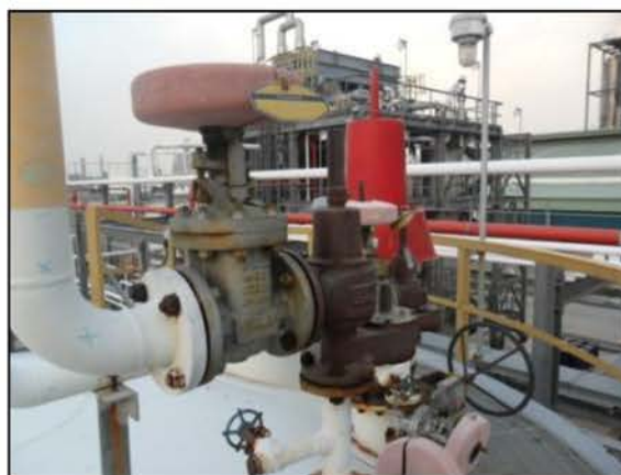
Pressure Vacuum Relief Valve
