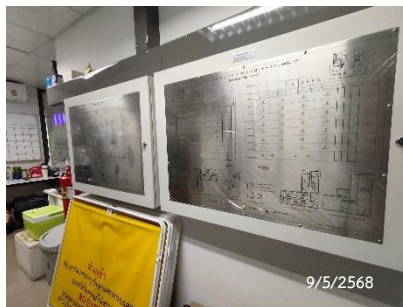
Graphic Annunciator Fire Alarm System
