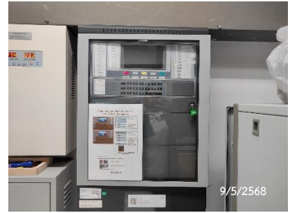
Fire Alarm Control Panel
