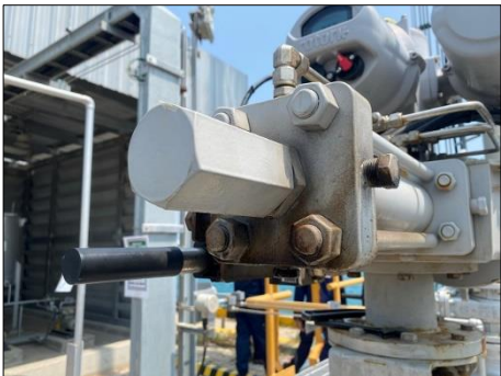
Fig 5. Was found oil leakage at end flange.
