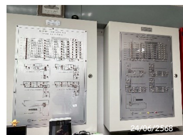
Graphic Annunciator Fire Alarm System
