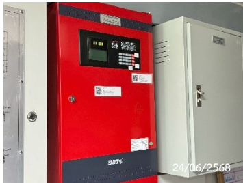
Fire Alarm Control Panel
