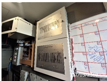
Graphic Annunciator Fire Alarm System
