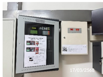
Fire Alarm Control Panel
