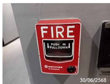
Fire Alarm Manual Station
