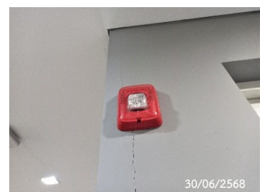
Indoor Selectable Output Speaker
