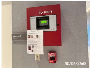
Fire Alarm Control Panel
