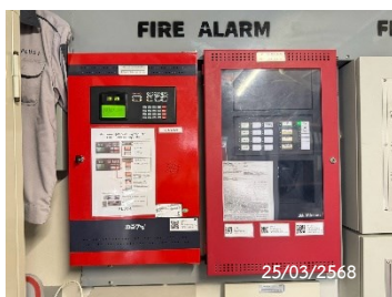
Fire Alarm Control Panel
