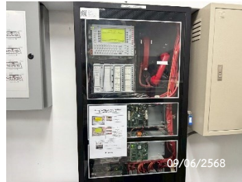
Fire Alarm Control Panel
