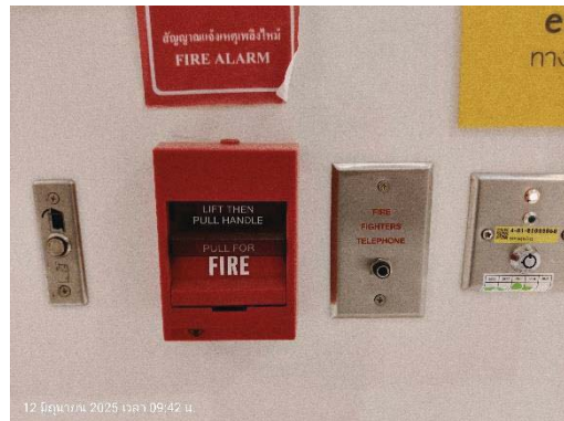
Fire Alarm Manual Station
