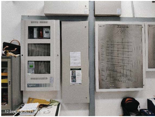
Fire Alarm Control Panel
