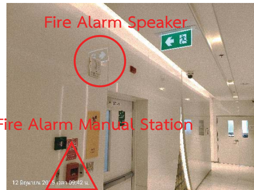
Fire Alarm Speaker & Fire Alarm Manual Station
