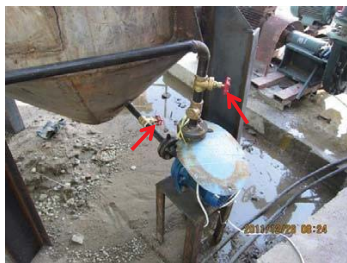
3. Check make-up water pump *Open valves
