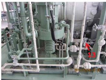
8. Open casing drain valve (13)
