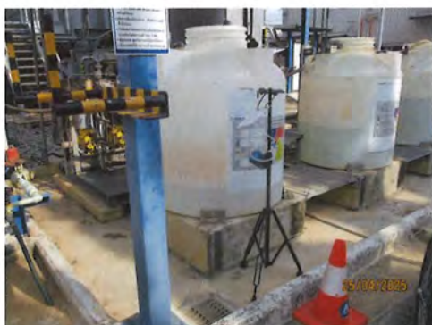
Sodium hydroxide tank (Boiler)
