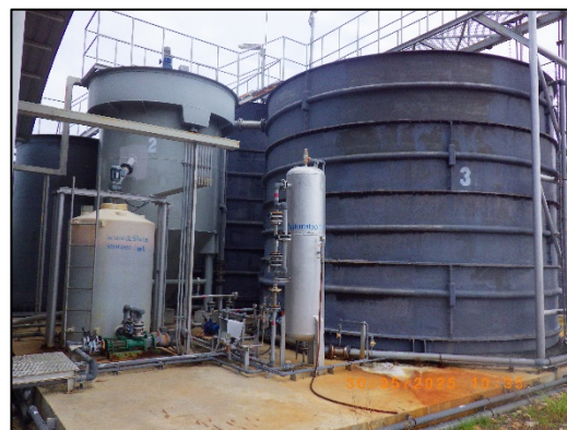
Dissolved Air Flotation (DAF)
