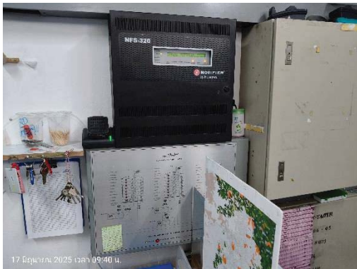
Fire Alarm Control Panel : FCP
