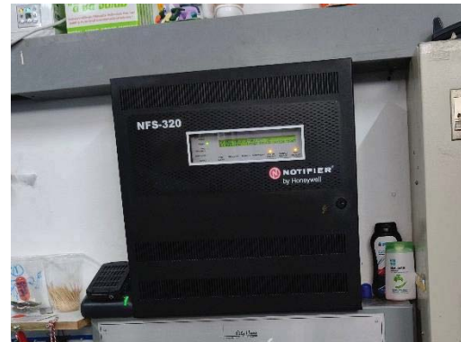
Fire Alarm Control Panel : FCP
