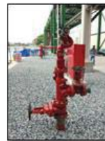
● Fire Hydrant with Monitor
