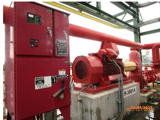
Electrical Driven Fire Water Pump
