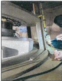
Figure 128.129: Connect of terminal main exciter
