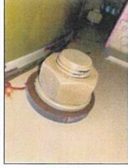
Figure 13: Through Bolt
