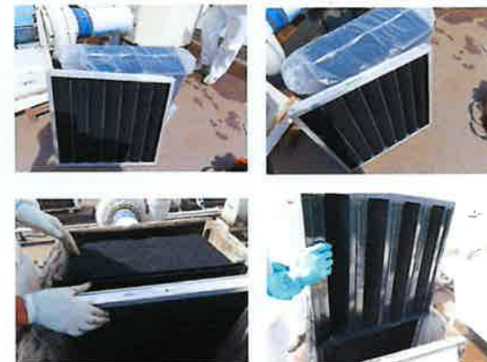
pre-filter and filter (after changing)
