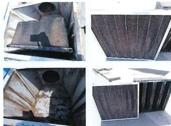
pre-filter and filter (before changing)
