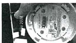
FL20 ROOM 2008 TEST SMOKE DETECTOR 1 SET...TROUBLE
