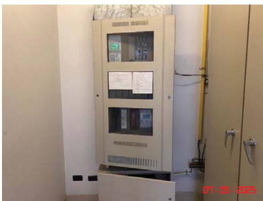
Fire Alarm Control Panel
