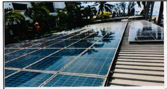
Description Cleaning PV-MT
