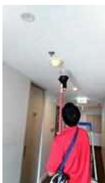
FL 18 IN FRONT OF LIFT SERVICE TEST SMOKE DETECTOR 1 SET
