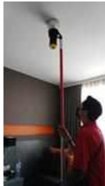
FL 22 ROOM 2216 SERVICE TEST SMOKE DETECTOR 1 SET
