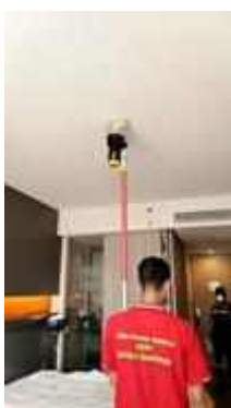
FL 22 ROOM 2220 TEST SMOKE DETECTOR 1 SET..NORMAL
