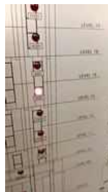
FL 14 ROOM 1423 TEST SMOKE DETECTOR 1 SET..NORMAL
