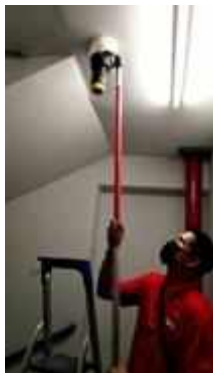
FL 18 FIRE ESCAPE SERVICE TEST SMOKE DETECTOR 1 SET
