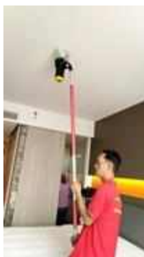
FL 22 ROOM 2208 TEST SMOKE DETECTOR 1 SET..NORMAL
