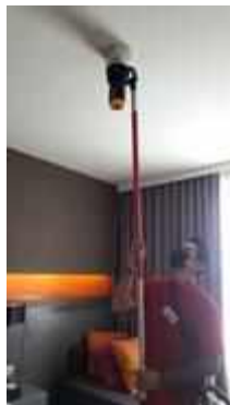
FL 21 ROOM 2112 SERVICE TEST SMOKE DETECTOR 1 SET
