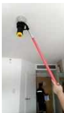
FL 15 ROOM 1522 TEST SMOKE DETECTOR 1 SET..NORMAL
