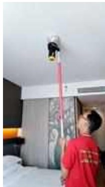
FL 23 ROOM 2305 TEST SMOKE DETECTOR 1 SET..NORMAL
