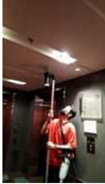
FL 18 CUSTOMER ELEVATOR FRONT SERVICE TEST SMOKE DETECTOR 1 SET
