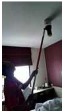
FL 10 ROOM 1010 TEST SMOKE DETECTOR 1 SET..NORMAL
