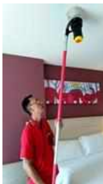
FL 15 ROOM 1517 TEST SMOKE DETECTOR 1 SET..NORMAL
