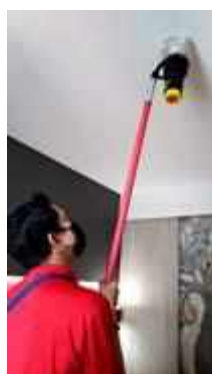
FL 24 ROOM 2419 SERVICE TEST SMOKE DETECTOR 1 SET
