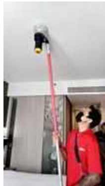
FL 26 ROOM 2605 SERVICE TEST SMOKE DETECTOR 1 SET
