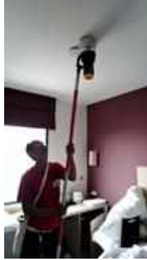
FL 10 ROOM 1004 TEST SMOKE DETECTOR 1 SET..NORMAL
