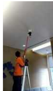
FL 21 ROOM 2118 SERVICE TEST SMOKE DETECTOR 1 SET
