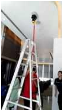
FL 9 GUEST ELEVATOR FRONT SERVICE TEST SMOKE DETECTOR 1 SET
