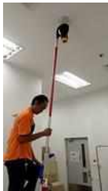
FL 7 TRAINING ROOM SERVICE TEST SMOKE DETECTOR 1 SET
