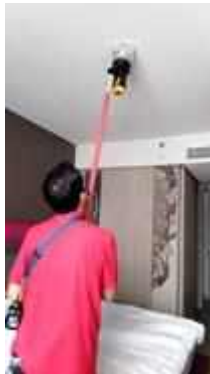
FL 27 ROOM 2711 SERVICE TEST SMOKE DETECTOR 1 SET
