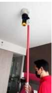
FL 26 ROOM 2610 SERVICE TEST SMOKE DETECTOR 1 SET
