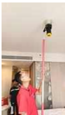
FL 26 ROOM 2620 TEST SMOKE DETECTOR 1 SET..NORMAL
