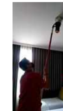
FL 27 ROOM 2701 SERVICE TEST SMOKE DETECTOR 1 SET
