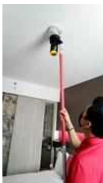
FL 27 ROOM 2706 SERVICE TEST SMOKE DETECTOR 1 SET
