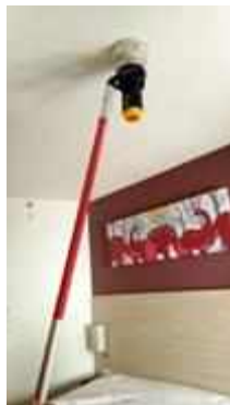
FL 11 ROOM 1107 TEST SMOKE DETECTOR 1 SET..NORMAL
