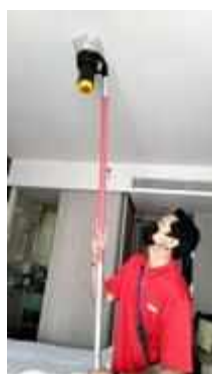
FL 22 ROOM 2209 SERVICE TEST SMOKE DETECTOR 1 SET
