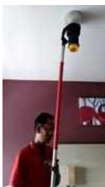
FL 15 ROOM 1524 TEST SMOKE DETECTOR 1 SET..NORMAL
