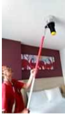
FL 14 ROOM 1417 TEST SMOKE DETECTOR 1 SET..NORMAL
