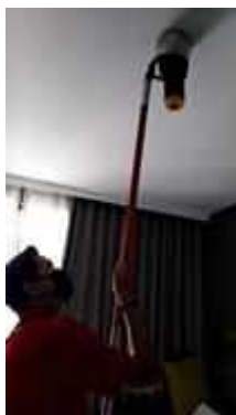
FL 18 ROOM 1801 SERVICE TEST SMOKE DETECTOR 1 SET
