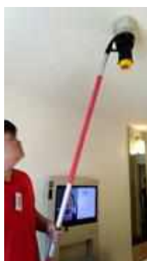
FL 14 ROOM 1424 TEST SMOKE DETECTOR 1 SET..NORMAL
