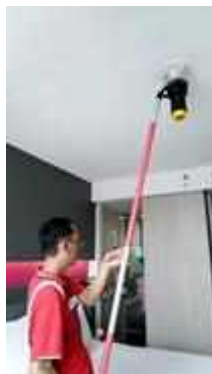
FL 24 ROOM 2417 TEST SMOKE DETECTOR 1 SET..NORMAL
