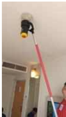
FL 17 ROOM 1725 TEST SMOKE DETECTOR 1 SET..NORMAL
