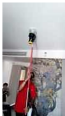
FL 24 ROOM 2414 SERVICE TEST SMOKE DETECTOR 1 SET
