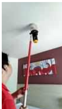
FL 11 ROOM 1103 TEST SMOKE DETECTOR 1 SET..NORMAL
