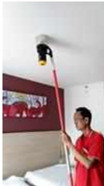
FL 16 ROOM 1608 TEST SMOKE DETECTOR 1 SET..NORMAL
