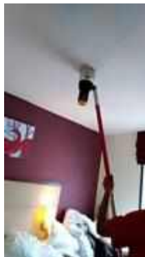
FL 10 ROOM 1011 TEST SMOKE DETECTOR 1 SET..NORMAL
