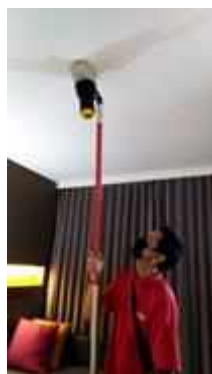
FL 22 ROOM 2212 SERVICE TEST SMOKE DETECTOR 1 SET
