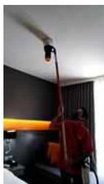
FL 22 ROOM 2206 SERVICE TEST SMOKE DETECTOR 1 SET
