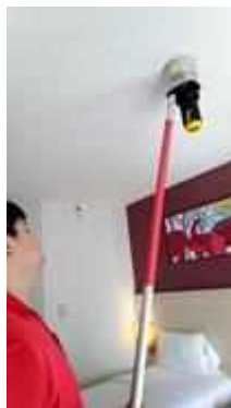
FL 15 ROOM 1528 TEST SMOKE DETECTOR 1 SET..NORMAL
