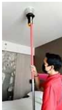
FL 25 ROOM 2508 SERVICE TEST SMOKE DETECTOR 1 SET
