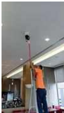
FL 21 ROOM 2118 SERVICE TEST SMOKE DETECTOR 1 SET
