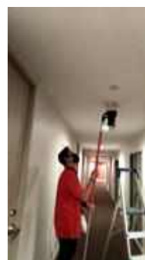
FL 18 IN FRONT OF LIFT SERVICE TEST SMOKE DETECTOR 1 SET
