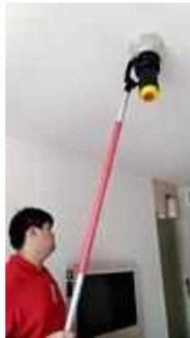
FL 14 ROOM 1421 TEST SMOKE DETECTOR 1 SET..NORMAL
