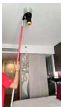
FL 26 ROOM 2604 SERVICE TEST SMOKE DETECTOR 1 SET
