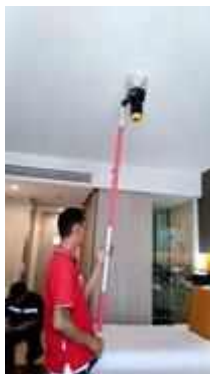
FL 23 ROOM 2302 TEST SMOKE DETECTOR 1 SET..NORMAL
