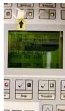
FL 16 ROOM 1623 TEST SMOKE DETECTOR 1 SET..NORMAL
