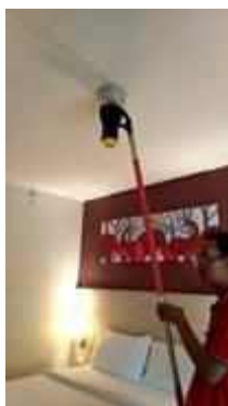
FL 14 ROOM 1403 TEST SMOKE DETECTOR 1 SET..NORMAL
