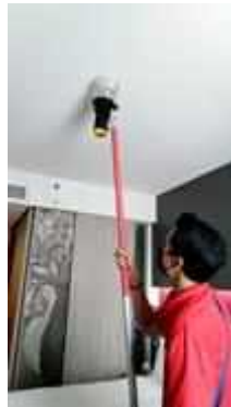
FL 25 ROOM 2510 SERVICE TEST SMOKE DETECTOR 1 SET
