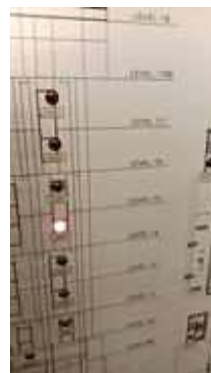
FL 14 ROOM 1414 TEST SMOKE DETECTOR 1 SET..NORMAL
