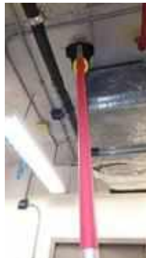
FL 18 PANTY ROOM TEST SMOKE DETECTOR 1 SET..NORMAL
