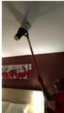
FL 12 ROOM 1207 TEST SMOKE DETECTOR 1 SET..NORMAL
