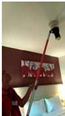
FL 17 ROOM 1705 TEST SMOKE DETECTOR 1 SET..NORMAL
