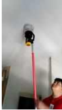
FL 12 ROOM 1212 TEST SMOKE DETECTOR 1 SET..NORMAL
