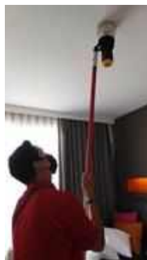
FL 22 ROOM 2201 SERVICE TEST SMOKE DETECTOR 1 SET
