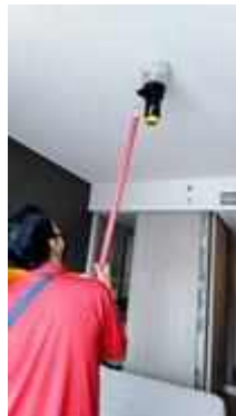
FL 23 ROOM 2307 SERVICE TEST SMOKE DETECTOR 1 SET
