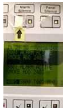
FL 24 ROOM 2402 TEST SMOKE DETECTOR 1 SET..NORMAL
