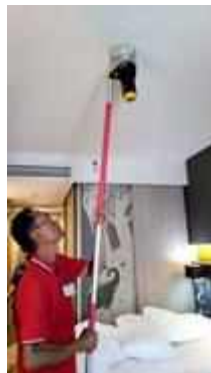
FL 19 ROOM 1912 TEST SMOKE DETECTOR 1 SET..NORMAL
