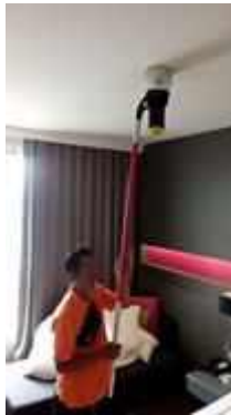
FL 25 ROOM 2505 SERVICE TEST SMOKE DETECTOR 1 SET
