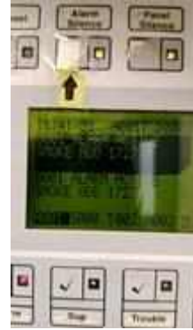
FL 17 ROOM 1727 TEST SMOKE DETECTOR 1 SET..NORMAL
