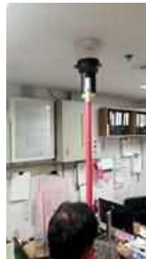
FL 7 ENGINEERING SERVICE TEST SMOKE DETECTOR 2 SET
