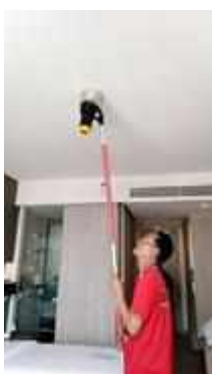
FL 22 ROOM 2202 TEST SMOKE DETECTOR 1 SET..NORMAL
