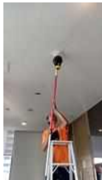
FL 21 ROOM 2118 SERVICE TEST SMOKE DETECTOR 1 SET
