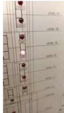
FL 14 ROOM 1421 TEST SMOKE DETECTOR 1 SET..NORMAL
