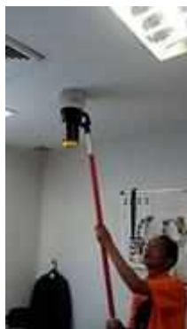
FL 7 HOUSEKEEPING SERVICE TEST SMOKE DETECTOR 2 SET
