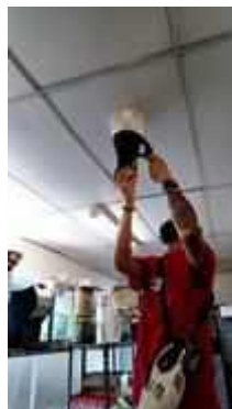
FL 8 EQUIPMENT STORAGE SERVICE TEST SMOKE DETECTOR 1 SET
