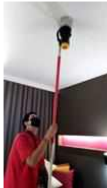
FL 27 ROOM 2709 SERVICE TEST SMOKE DETECTOR 1 SET
