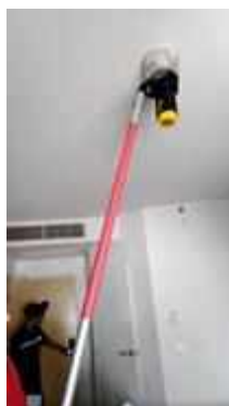
FL 15 ROOM 1520 TEST SMOKE DETECTOR 1 SET..NORMAL
