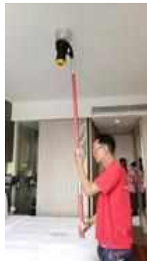
FL 19 ROOM 1911 TEST SMOKE DETECTOR 1 SET..NORMAL
