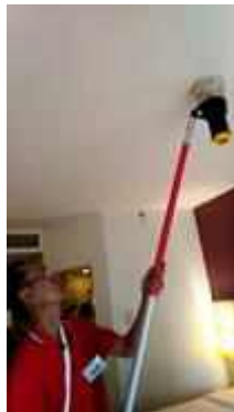
FL 10 ROOM 1028 TEST SMOKE DETECTOR 1 SET..NORMAL
