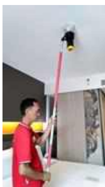
FL 22 ROOM 2211 TEST SMOKE DETECTOR 1 SET..NORMAL
