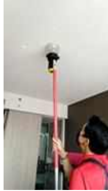
FL 27 ROOM 2708 SERVICE TEST SMOKE DETECTOR 1 SET
