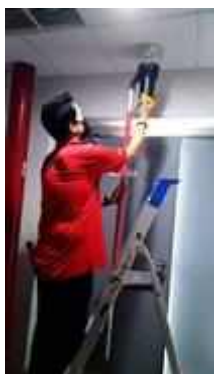
FL 18 IN FRONT OF LIFT SERVICE TEST SMOKE DETECTOR 1 SET
