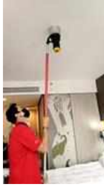
FL 19 ROOM 1902 SERVICE TEST SMOKE DETECTOR 1 SET
