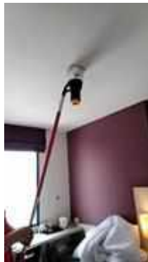
FL 10 ROOM 1017 TEST SMOKE DETECTOR 1 SET..NORMAL
