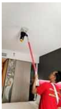
FL 24 ROOM 2406 TEST SMOKE DETECTOR 1 SET..NORMAL
