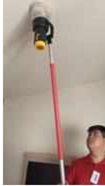
FL 16 ROOM 1604 TEST SMOKE DETECTOR 1 SET..NORMAL
