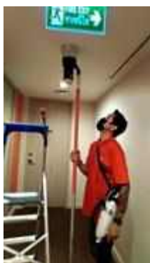
FL 18 CORRIDOR SERVICE TEST SMOKE DETECTOR 5 SET
