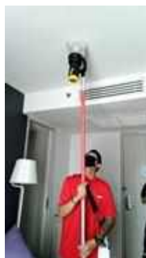
FL 24 ROOM 2414 SERVICE TEST SMOKE DETECTOR 1 SET
