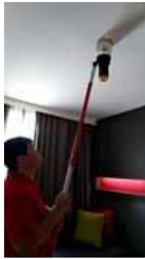
FL 28 ROOM 2811 TEST SMOKE DETECTOR 1 SET..NORMAL
