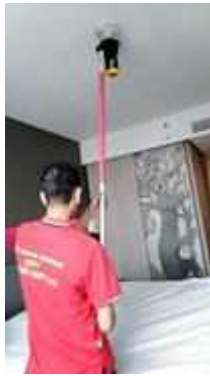
FL 18 ROOM 1815 TEST SMOKE DETECTOR 1 SET..NORMAL
