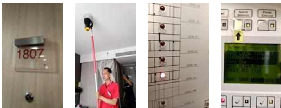
FL 18 ROOM 1807 TEST SMOKE DETECTOR 1 SET..NORMAL
