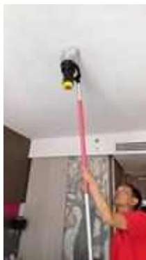
FL 24 ROOM 2401 TEST SMOKE DETECTOR 1 SET..NORMAL
