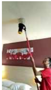
FL 12 ROOM 1216 TEST SMOKE DETECTOR 1 SET..NORMAL
