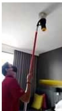
FL 19 ROOM 1909 SERVICE TEST SMOKE DETECTOR 1 SET
