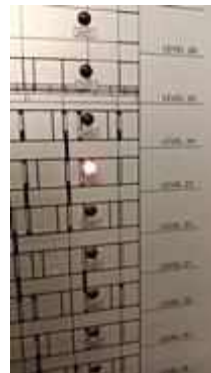
FL 23 ROOM 2319 TEST SMOKE DETECTOR 1 SET..NORMAL
