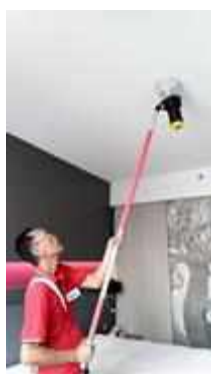
FL 24 ROOM 2405 TEST SMOKE DETECTOR 1 SET..NORMAL
