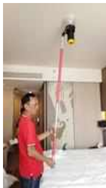
FL 18 ROOM 1805 TEST SMOKE DETECTOR 1 SET..NORMAL
