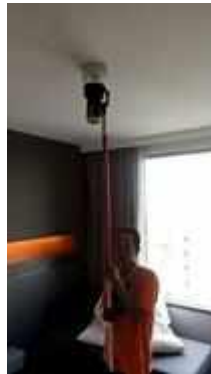
FL 21 ROOM 2120 SERVICE TEST SMOKE DETECTOR 1 SET
