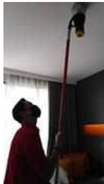
FL 21 ROOM 2101 SERVICE TEST SMOKE DETECTOR 1 SET
