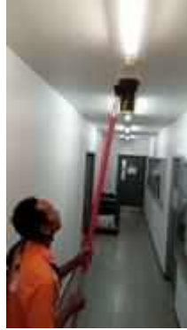
FL 8 CORRIDOR SERVICE TEST SMOKE DETECTOR 6 SET
