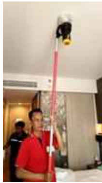
FL 23 ROOM 2304 TEST SMOKE DETECTOR 1 SET..NORMAL
