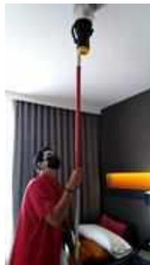
FL 23 ROOM 2301 SERVICE TEST SMOKE DETECTOR 1 SET
