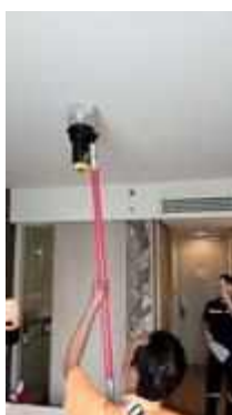
FL 27 ROOM 2707 SERVICE TEST SMOKE DETECTOR 1 SET
