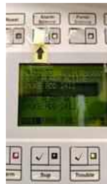
FL 23 ROOM 2302 TEST SMOKE DETECTOR 1 SET..NORMAL
