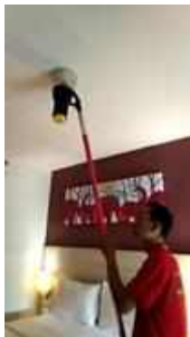
FL 17 ROOM 1709 TEST SMOKE DETECTOR 1 SET..NORMAL
