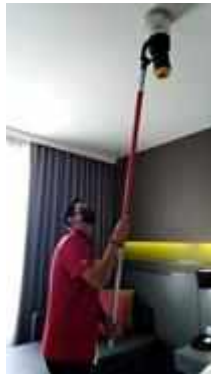
FL 20 ROOM 2005 SERVICE TEST SMOKE DETECTOR 1 SET
