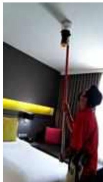
FL 19 ROOM 1910 SERVICE TEST SMOKE DETECTOR 1 SET
