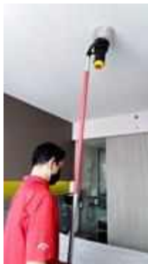
FL 20 ROOM 2019 SERVICE TEST SMOKE DETECTOR 1 SET
