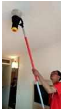
FL 17 ROOM 1702 TEST SMOKE DETECTOR 1 SET..NORMAL
