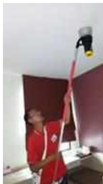
FL 12 ROOM 1208 TEST SMOKE DETECTOR 1 SET..NORMAL
