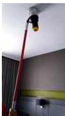
FL 19 ROOM 1901 SERVICE TEST SMOKE DETECTOR 1 SET
