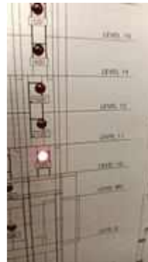
FL 10 ROOM 1028 TEST SMOKE DETECTOR 1 SET..NORMAL
