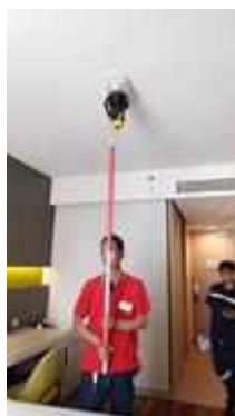
FL 18 ROOM 1804 TEST SMOKE DETECTOR 1 SET..NORMAL
