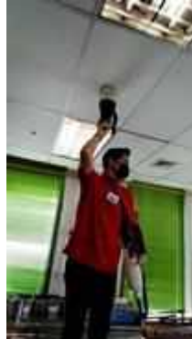
FL 8 CANTEEN SERVICE TEST SMOKE DETECTOR 2 SET NOWORK
