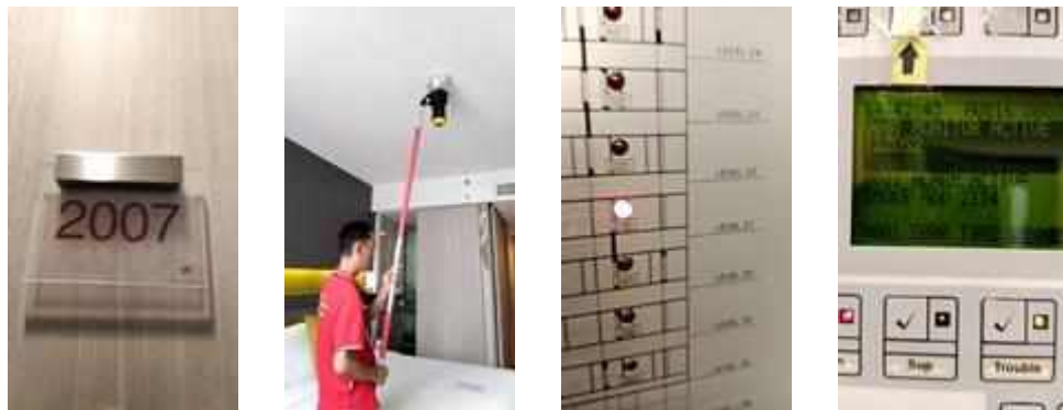
FL 20 ROOM 2007 TEST SMOKE DETECTOR 1 SET..NORMAL
