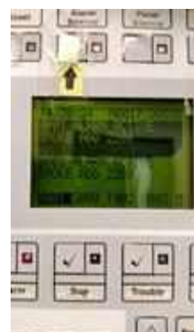
FL 22 ROOM 2211 TEST SMOKE DETECTOR 1 SET..NORMAL
