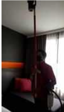
FL 21 ROOM 2108 SERVICE TEST SMOKE DETECTOR 1 SET
