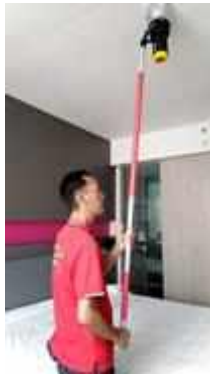
FL 28 ROOM 2818 TEST SMOKE DETECTOR 1 SET..NORMAL
