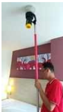
FL 11 ROOM 1118 TEST SMOKE DETECTOR 1 SET..NORMAL
