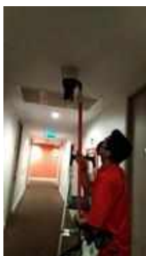
FL 18 CORRIDOR SERVICE TEST SMOKE DETECTOR 5 SET
