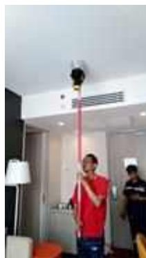
FL 23 ROOM 2314 TEST SMOKE DETECTOR 1 SET..NORMAL
