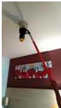
FL 16 ROOM 1609 TEST SMOKE DETECTOR 1 SET..NORMAL
