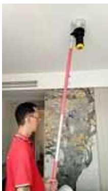
FL 22 ROOM 2218 TEST SMOKE DETECTOR 1 SET..NORMAL
