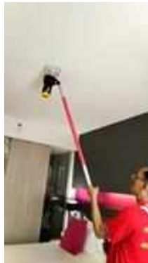
FL 28 ROOM 2804 TEST SMOKE DETECTOR 1 SET..NORMAL
