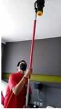
FL 20 ROOM 2017 SERVICE TEST SMOKE DETECTOR 1 SET
