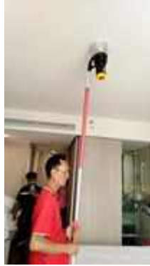
FL 21 ROOM 2104 TEST SMOKE DETECTOR 1 SET..NORMAL
