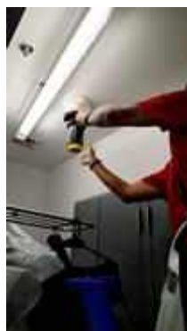
FL 9 EXECUTIVE OFFICE SERVICE TEST SMOKE DETECTOR 5 SET
