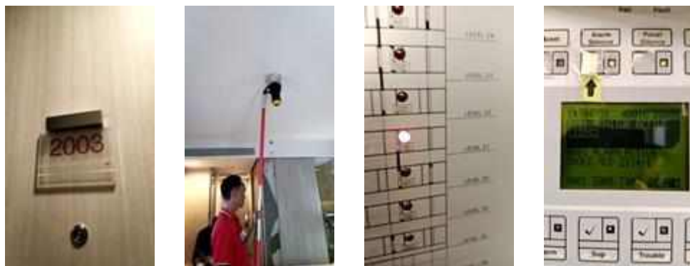
FL 20 ROOM 2003 TEST SMOKE DETECTOR 1 SET..NORMAL
