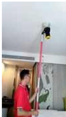
FL 19 ROOM 1905 TEST SMOKE DETECTOR 1 SET..NORMAL
