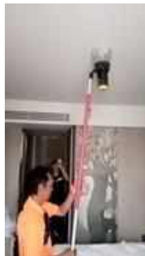
FL 25 ROOM 2503 SERVICE TEST SMOKE DETECTOR 1 SET
