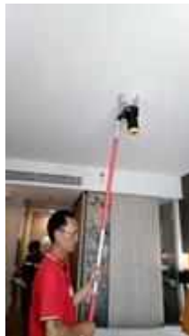
FL 20 ROOM 2002 TEST SMOKE DETECTOR 1 SET..NORMAL
