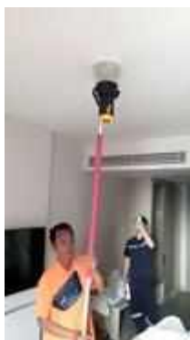
FL 28 ROOM 2812 SERVICE TEST SMOKE DETECTOR 1 SET
