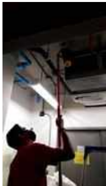
FL 18 MAID'S ROOM SERVICE TEST SMOKE DETECTOR 1 SET
