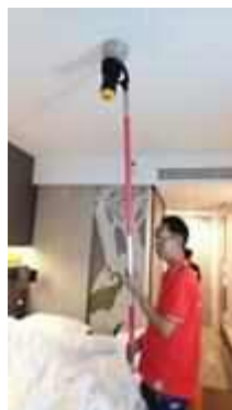
FL 19 ROOM 1917 TEST SMOKE DETECTOR 1 SET..NORMAL
