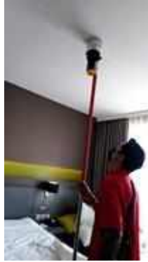
FL 18 ROOM 1802 SERVICE TEST SMOKE DETECTOR 1 SET
