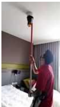
FL 18 ROOM 1810 SERVICE TEST SMOKE DETECTOR 1 SET GRAPHIC AT 1811 AD3911607702
