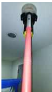
FL 17 PANTY ROOM TEST SMOKE DETECTOR 1 SET..NORMAL
