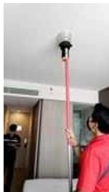
FL 26 ROOM 2610 SERVICE TEST SMOKE DETECTOR 1 SET
