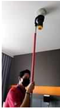
FL 21 ROOM 2105 SERVICE TEST SMOKE DETECTOR 1 SET
