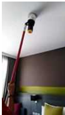
FL 18 ROOM 1809 SERVICE TEST SMOKE DETECTOR 1 SET
