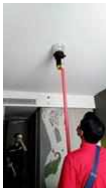
FL 19 ROOM 1904 SERVICE TEST SMOKE DETECTOR 1 SET
