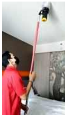
FL 23 ROOM 2317 SERVICE TEST SMOKE DETECTOR 1 SET
