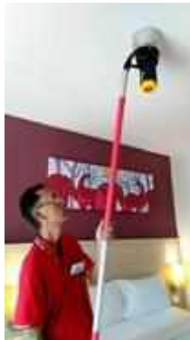
FL 15 ROOM 1515 TEST SMOKE DETECTOR 1 SET..NORMAL
