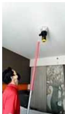
FL 23 ROOM 2318 SERVICE TEST SMOKE DETECTOR 1 SET
