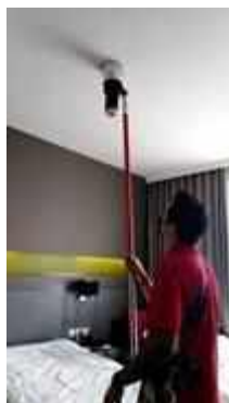
FL 20 ROOM 2004 SERVICE TEST SMOKE DETECTOR 1 SET
