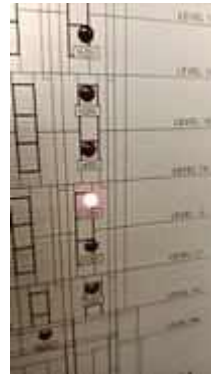
FL 12 ROOM 1207 TEST SMOKE DETECTOR 1 SET..NORMAL
