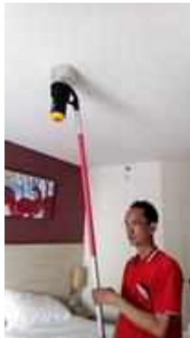
FL 14 ROOM 1427 TEST SMOKE DETECTOR 1 SET..NORMAL
