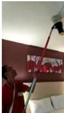
FL 15 ROOM 1505 TEST SMOKE DETECTOR 1 SET..NORMAL
