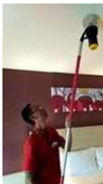
FL 14 ROOM 1404 TEST SMOKE DETECTOR 1 SET..NORMAL
