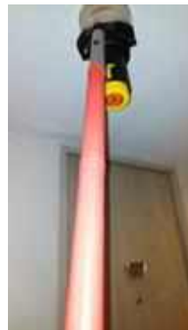
FL 18 PANTY ROOM TEST SMOKE DETECTOR 1 SET..NORMAL
