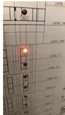
FL 17 ROOM 1726 TEST SMOKE DETECTOR 1 SET..NORMAL
