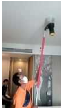
FL 25 ROOM 2506 SERVICE TEST SMOKE DETECTOR 1 SET
