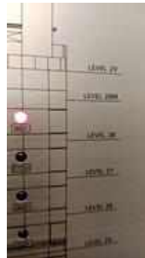
FL 28 ROOM 2807 TEST SMOKE DETECTOR 1 SET..NORMAL
