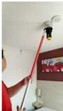
FL 10 ROOM 1001 TEST SMOKE DETECTOR 1 SET..NORMAL
