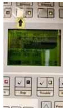
FL 16 ROOM 1602 TEST SMOKE DETECTOR 1 SET..NORMAL
