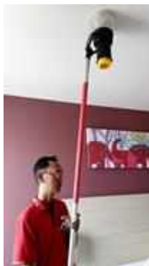
FL 12 ROOM 1205 TEST SMOKE DETECTOR 1 SET..NORMAL
