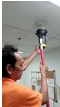
FL 7 ENGINEERING SERVICE TEST SMOKE DETECTOR 2 SET
