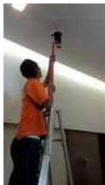
FL 8 RESTAURANT SERVICE TEST SMOKE DETECTOR 6 SET
