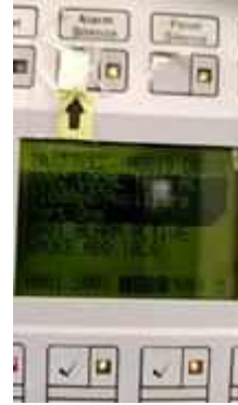
FL 11 ROOM 1122 TEST SMOKE DETECTOR 1 SET..NORMAL
