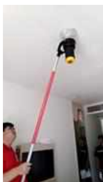
FL 16 ROOM 1603 TEST SMOKE DETECTOR 1 SET..NORMAL
