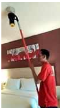
FL 16 ROOM 1621 TEST SMOKE DETECTOR 1 SET..NORMAL
