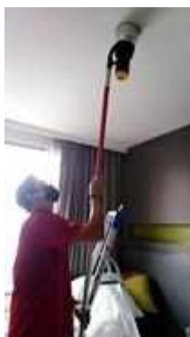
FL 18 ROOM 1811 SERVICE TEST SMOKE DETECTOR 1 SET GRAPHIC AT 1812 AD3911606941
