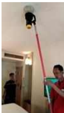
FL 10 ROOM 1024 TEST SMOKE DETECTOR 1 SET..NORMAL
