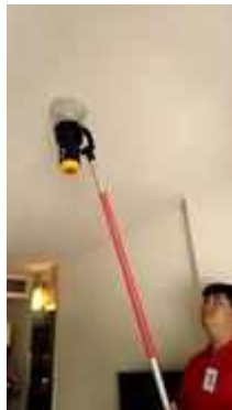
FL 11 ROOM 1112 TEST SMOKE DETECTOR 1 SET..NORMAL
