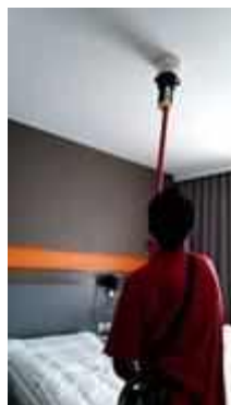
FL 21 ROOM 2103 SERVICE TEST SMOKE DETECTOR 1 SET
