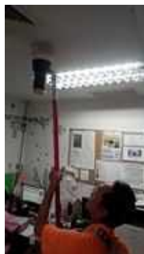
FL 7 HOUSEKEEPING SERVICE TEST SMOKE DETECTOR 2 SET
