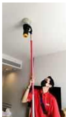
FL 25 ROOM 2507 SERVICE TEST SMOKE DETECTOR 1 SET
