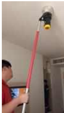
FL 1614 ROOM 1424 TEST SMOKE DETECTOR 1 SET..NORMAL
