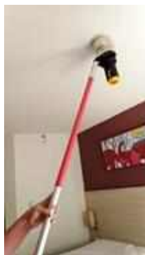
FL 11 ROOM 1126 TEST SMOKE DETECTOR 1 SET..NORMAL
