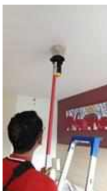
FL 16 ROOM 1623 TEST SMOKE DETECTOR 1 SET..NORMAL
