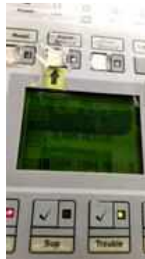
FL 7 IN FRONT OF LIFT SERVICE TEST SMOKE DETECTOR 1 SET
