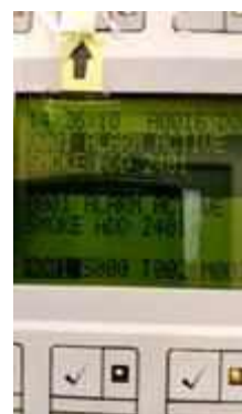
FL 24 ROOM 2403 TEST SMOKE DETECTOR 1 SET..NORMAL
