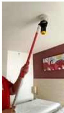
FL 11 ROOM 1116 TEST SMOKE DETECTOR 1 SET..NORMAL
