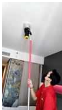
FL 27 ROOM 2720 SERVICE TEST SMOKE DETECTOR 1 SET
