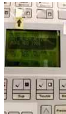
FL 19 ROOM 1917 TEST SMOKE DETECTOR 1 SET..NORMAL
