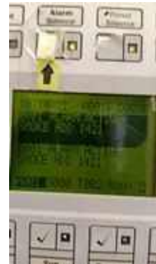
FL 15 ROOM 1527 TEST SMOKE DETECTOR 1 SET..NORMAL
