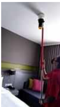
FL 20 ROOM 2008 SERVICE TEST SMOKE DETECTOR 1 SET
