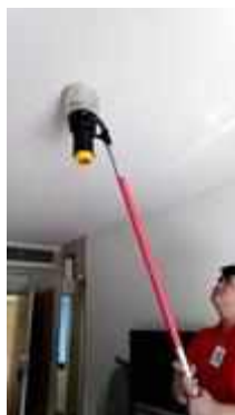
FL 10 ROOM 1002 TEST SMOKE DETECTOR 1 SET..NORMAL
