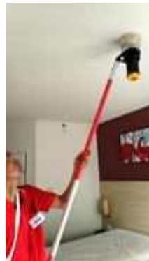
FL 11 ROOM 1128 TEST SMOKE DETECTOR 1 SET..NORMAL
