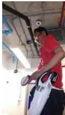
FL 18 PANTY ROOM TEST SMOKE DETECTOR 1 SET..NORMAL
