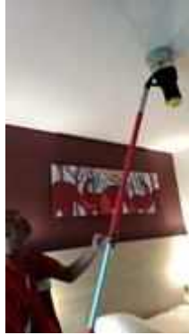
FL 17 ROOM 1710 TEST SMOKE DETECTOR 1 SET..NORMAL
