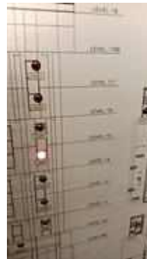
FL 15 ROOM 1505 TEST SMOKE DETECTOR 1 SET..NORMAL
