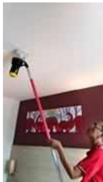
FL 17 ROOM 1721 TEST SMOKE DETECTOR 1 SET..NORMAL
