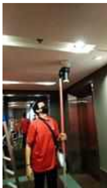
FL 19 CUSTOMER ELEVATOR FRONT SERVICE TEST SMOKE DETECTOR 1 SET
