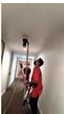
FL 18 IN FRONT OF LIFT SERVICE TEST SMOKE DETECTOR 1 SET
