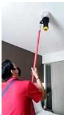
FL 27 ROOM 2702 SERVICE TEST SMOKE DETECTOR 1 SET
