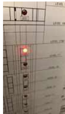
FL 17 ROOM 1725 TEST SMOKE DETECTOR 1 SET..NORMAL
