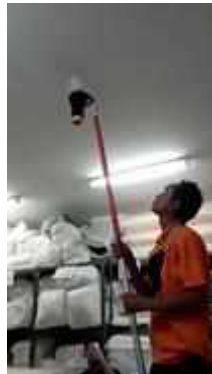
FL 7 CLEAN LINEN SERVICE TEST SMOKE DETECTOR 1 SET
