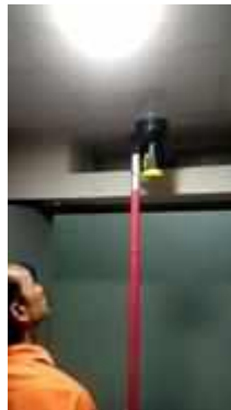
FL 7 IN FRONT OF LIFT SERVICE TEST SMOKE DETECTOR 1 SET
