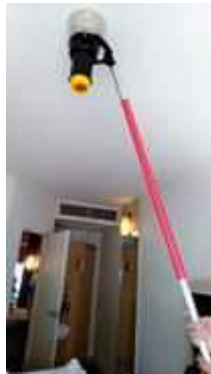
FL 15 ROOM 1527 TEST SMOKE DETECTOR 1 SET..NORMAL
