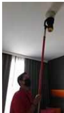
FL 22 ROOM 2219 SERVICE TEST SMOKE DETECTOR 1 SET
