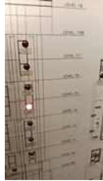
FL 14 ROOM 1417 TEST SMOKE DETECTOR 1 SET..NORMAL
