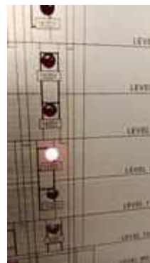
FL 12 ROOM 1211 TEST SMOKE DETECTOR 1 SET..NORMAL
