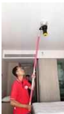
FL 24 ROOM 2402 TEST SMOKE DETECTOR 1 SET..NORMAL
