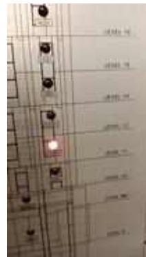
FL 11 ROOM 1106 TEST SMOKE DETECTOR 1 SET..NORMAL
