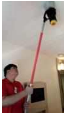
FL 12 ROOM 1218 TEST SMOKE DETECTOR 1 SET..NORMAL
