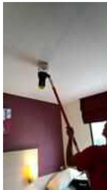
FL 10 ROOM 1009 TEST SMOKE DETECTOR 1 SET..NORMAL
