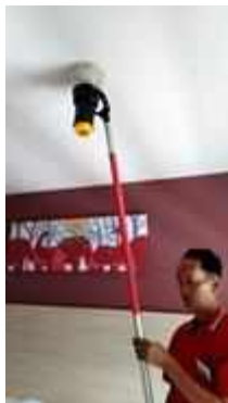
FL 10 ROOM 1021 TEST SMOKE DETECTOR 1 SET..NORMAL
