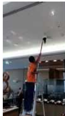
FL 21 ROOM 2118 SERVICE TEST SMOKE DETECTOR 1 SET
