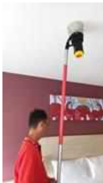
FL 11 ROOM 1104 TEST SMOKE DETECTOR 1 SET..NORMAL
