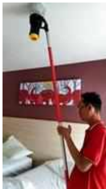
FL 12 ROOM 1226 TEST SMOKE DETECTOR 1 SET..NORMAL
