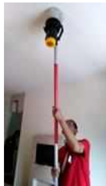
FL 12 ROOM 1224 TEST SMOKE DETECTOR 1 SET..NORMAL
