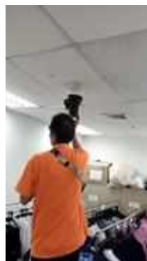
FL 7 UNIFORM SERVICE TEST SMOKE DETECTOR 1 SET NOWORK
