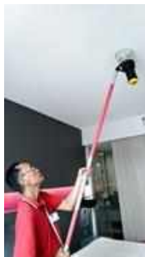
FL 28 ROOM 2809 TEST SMOKE DETECTOR 1 SET..NORMAL
