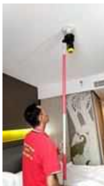
FL 23 ROOM 2314 TEST SMOKE DETECTOR 1 SET..NORMAL
