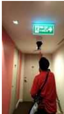
FL 19 CORRIDOR SERVICE TEST SMOKE DETECTOR 5 SET
