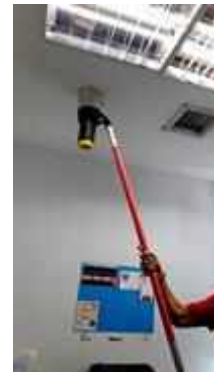
FL 9 GUEST LUGGAGE STORAGE ROOM ELEVATOR FRONT SERVICE TEST SMOKE DETECTOR 1 SET
