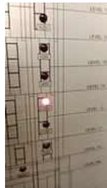
FL 12 ROOM 1224 TEST SMOKE DETECTOR 1 SET..NORMAL
