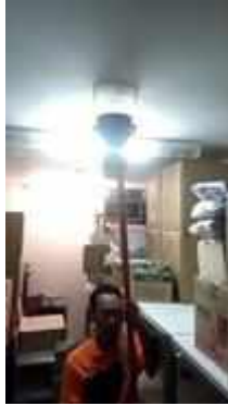
FL 7 STORGE SERVICE TEST SMOKE DETECTOR 1 SET
