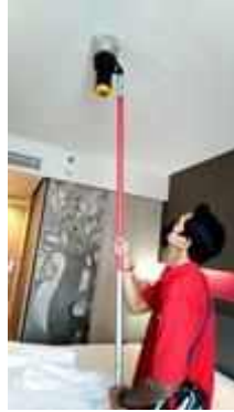
FL 24 ROOM 2420 SERVICE TEST SMOKE DETECTOR 1 SET
