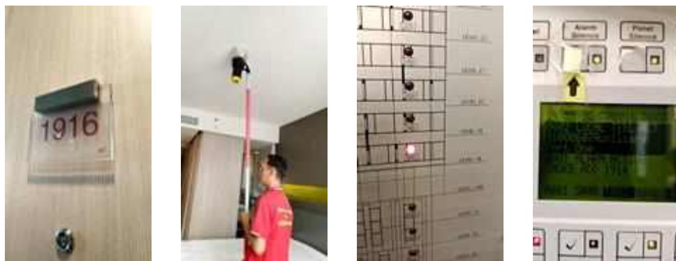
FL 19 ROOM 1916 TEST SMOKE DETECTOR 1 SET..NORMAL
