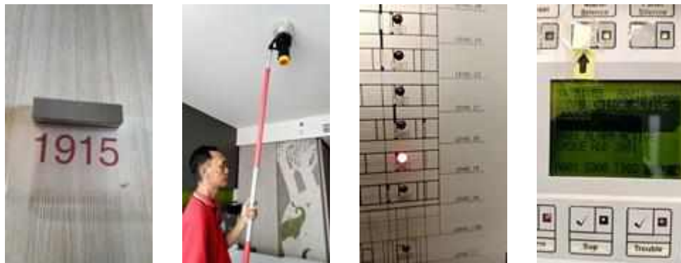
FL 19 ROOM 1915 TEST SMOKE DETECTOR 1 SET..NORMAL
