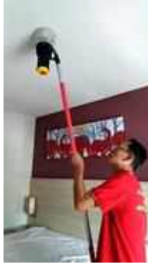
FL 10 ROOM 1006 TEST SMOKE DETECTOR 1 SET..NORMAL
