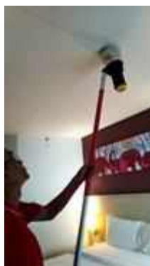
FL 12 ROOM 1209 TEST SMOKE DETECTOR 1 SET..NORMAL
