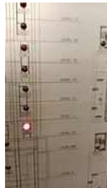
FL 10 ROOM 1003 TEST SMOKE DETECTOR 1 SET..NORMAL
