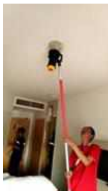
FL 17 ROOM 1708 TEST SMOKE DETECTOR 1 SET..NORMAL
