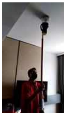
FL 22 ROOM 2214 SERVICE TEST SMOKE DETECTOR 2 SET
