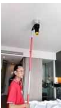
FL 22 ROOM 2201 TEST SMOKE DETECTOR 1 SET..NORMAL
