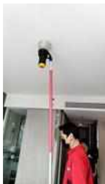
FL 19 ROOM 1919 SERVICE TEST SMOKE DETECTOR 1 SE
