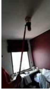
FL 11 ROOM 1105 TEST SMOKE DETECTOR 1 SET..NORMAL
