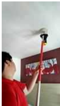
FL 12 ROOM 1206 TEST SMOKE DETECTOR 1 SET..NORMAL
