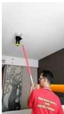
FL 23 ROOM 2303 TEST SMOKE DETECTOR 1 SET..NORMAL
