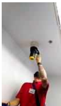
FL 9 EXECUTIVE OFFICE SERVICE TEST SMOKE DETECTOR 5 SET
