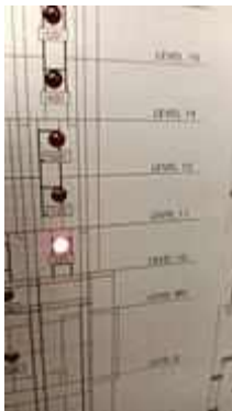
FL 10 ROOM 1011 TEST SMOKE DETECTOR 1 SET..NORMAL
