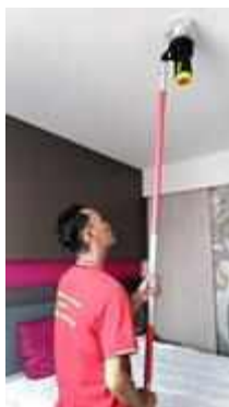
FL 28 ROOM 2805 TEST SMOKE DETECTOR 1 SET..NORMAL
