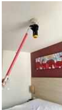
FL 11 ROOM 1106 TEST SMOKE DETECTOR 1 SET..NORMAL
