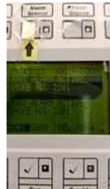
FL 19 ROOM 1911 TEST SMOKE DETECTOR 1 SET..NORMAL
