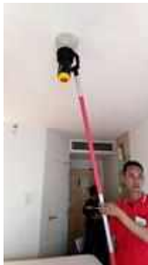
FL 10 ROOM 1027 TEST SMOKE DETECTOR 1 SET..NORMAL
