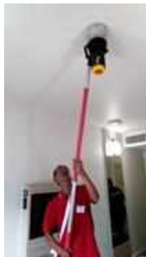
FL 15 ROOM 1506 TEST SMOKE DETECTOR 1 SET..NORMAL
