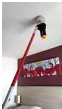
FL 12 ROOM 1211 TEST SMOKE DETECTOR 1 SET..NORMAL
