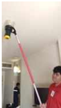
FL 16 ROOM 1615 TEST SMOKE DETECTOR 1 SET..NORMAL
