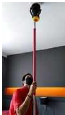
FL 21 ROOM 2117 SERVICE TEST SMOKE DETECTOR 1 SET
