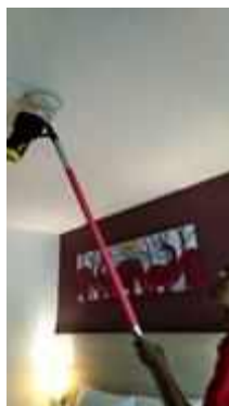
FL 14 ROOM 1414 TEST SMOKE DETECTOR 1 SET..NORMAL
