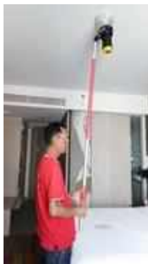
FL 28 ROOM 2801 TEST SMOKE DETECTOR 1 SET..NORMAL
