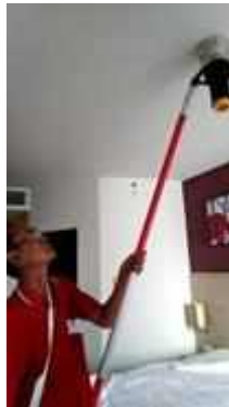
FL 16 ROOM 1611 TEST SMOKE DETECTOR 1 SET..NORMAL
