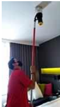
FL 19 ROOM 1907 SERVICE TEST SMOKE DETECTOR 1 SET
