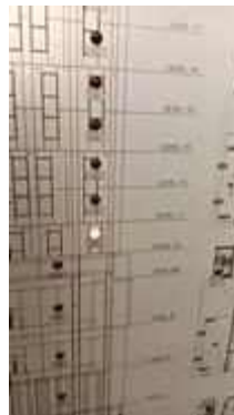
FL 12 ROOM 1219 TEST SMOKE DETECTOR 1 SET..NORMAL
