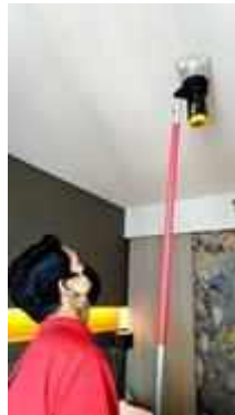
FL 21 ROOM 2119 SERVICE TEST SMOKE DETECTOR 1 SET
