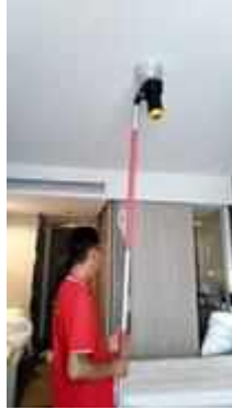
FL 19 ROOM 1908 TEST SMOKE DETECTOR 1 SET..NORMAL
