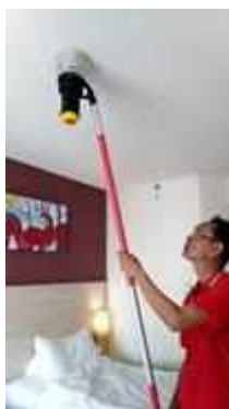
FL 14 ROOM 1425 TEST SMOKE DETECTOR 1 SET..NORMAL
