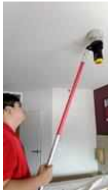
FL 15 ROOM 1523 TEST SMOKE DETECTOR 1 SET..NORMAL
