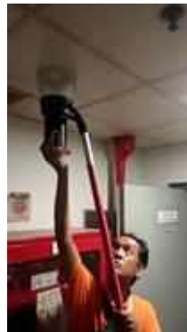
FL 1 IN FRONT OF LIFT SERVICE TEST SMOKE DETECTOR 1 SET
