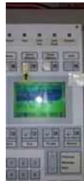
FL 23 ROOM 2317 SERVICE TEST SMOKE DETECTOR 1 SET
