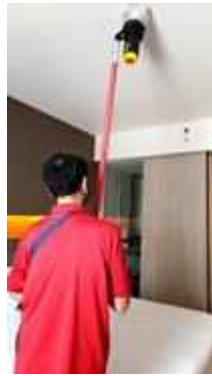
FL 23 ROOM 2315 SERVICE TEST SMOKE DETECTOR 1 SET
