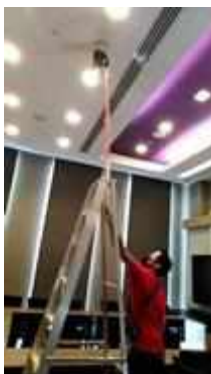
FL 9 SIAM ROOM SERVICE TEST SMOKE DETECTOR 1 SET
