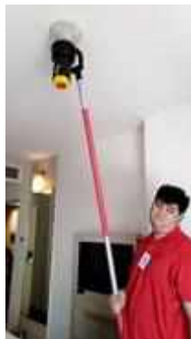
FL 12 ROOM 1225 TEST SMOKE DETECTOR 1 SET..NORMAL
