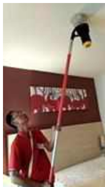
FL 16 ROOM 1612 TEST SMOKE DETECTOR 1 SET..NORMAL
