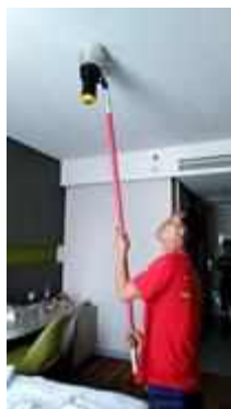
FL 19 ROOM 1906 TEST SMOKE DETECTOR 1 SET..NORMAL
