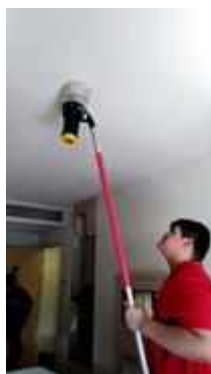
FL 14 ROOM 1423 TEST SMOKE DETECTOR 1 SET..NORMAL
