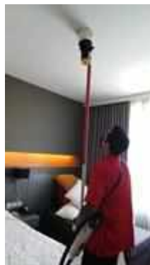
FL 21 ROOM 2116 SERVICE TEST SMOKE DETECTOR 1 SET
