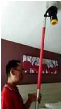
FL 12 ROOM 1219 TEST SMOKE DETECTOR 1 SET..NORMAL
