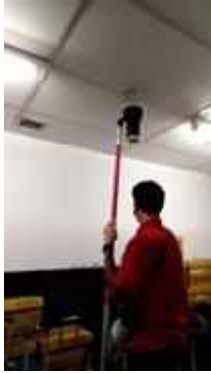
FL 9 GUEST LUGGAGE STORAGE ROOM ELEVATOR FRONT SERVICE TEST SMOKE DETECTOR 1 SET
