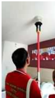
FL 10 ROOM 1003 TEST SMOKE DETECTOR 1 SET..NORMAL
