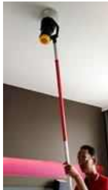
FL 24 ROOM 2404 TEST SMOKE DETECTOR 1 SET..NORMAL
