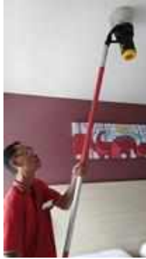
FL 11 ROOM 1122 TEST SMOKE DETECTOR 1 SET..NORMAL
