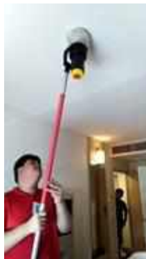
FL 12 ROOM 1221 TEST SMOKE DETECTOR 1 SET..NORMAL
