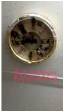
FL 1 RECYCLE GARBAGE SMOKE DETECTOR 1 SET NOWORK
