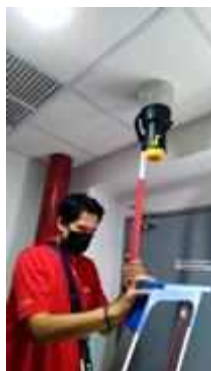
FL 19 IN FRONT OF LIFT SERVICE TEST SMOKE DETECTOR 1 SET
