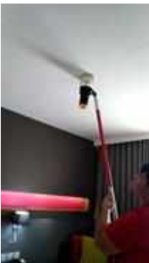
FL 28 ROOM 2808 TEST SMOKE DETECTOR 1 SET.. NOWORK
