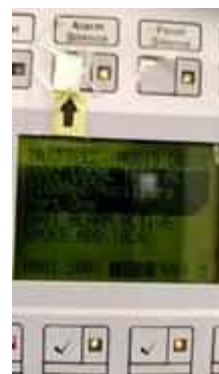
FL 14 ROOM 1403 TEST SMOKE DETECTOR 1 SET..NORMAL
