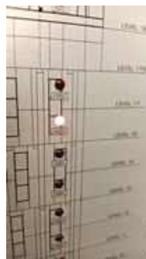
FL 16 ROOM 1621 TEST SMOKE DETECTOR 1 SET..NORMAL
