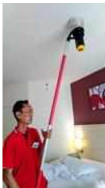
FL 14 ROOM 1426 TEST SMOKE DETECTOR 1 SET..NORMAL
