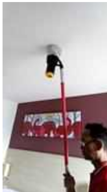
FL 11 ROOM 1101 TEST SMOKE DETECTOR 1 SET..NORMAL
