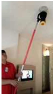
FL 11 ROOM 1120 TEST SMOKE DETECTOR 1 SET..NORMAL
