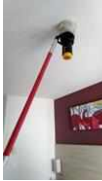
FL 11 ROOM 1109 TEST SMOKE DETECTOR 1 SET..NORMAL
