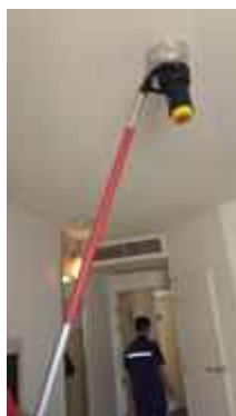
FL 16 ROOM 1601 TEST SMOKE DETECTOR 1 SET..NORMAL
