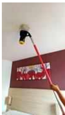
FL 17 ROOM 1707 TEST SMOKE DETECTOR 1 SET..NORMAL
