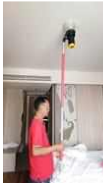
FL 18 ROOM 1812 TEST SMOKE DETECTOR 1 SET..NORMAL
