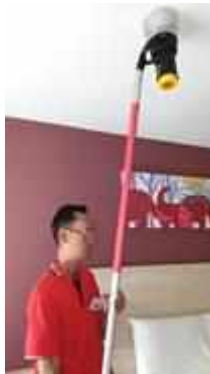
FL 12 ROOM 1215 TEST SMOKE DETECTOR 1 SET..NORMAL
