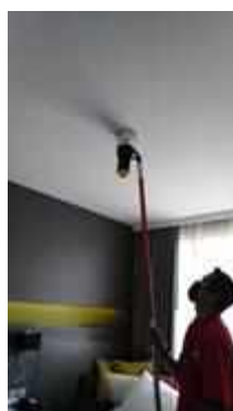
FL 20 ROOM 2010 SERVICE TEST SMOKE DETECTOR 1 SET
