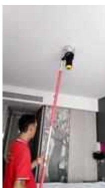
FL 24 ROOM 2403 TEST SMOKE DETECTOR 1 SET..NORMAL
