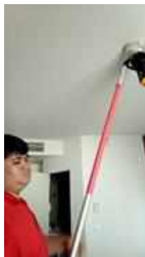
FL 14 ROOM 1420 TEST SMOKE DETECTOR 1 SET..NORMAL
