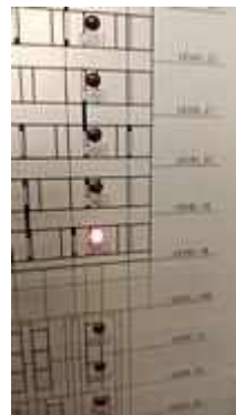
FL 18 ROOM 1805 TEST SMOKE DETECTOR 1 SET..NORMAL
