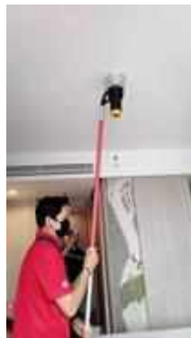
FL 18 ROOM 1806 SERVICE TEST SMOKE DETECTOR 1 SET
