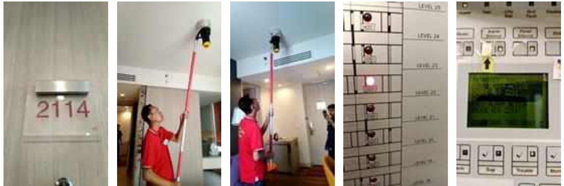
FL 21 ROOM 2114 TEST SMOKE DETECTOR 2 SET..NORMAL
