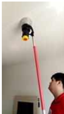
FL 11 ROOM 1102 TEST SMOKE DETECTOR 1 SET..NORMAL
