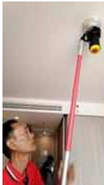
FL 24 ROOM 2412 TEST SMOKE DETECTOR 1 SET..NORMAL
