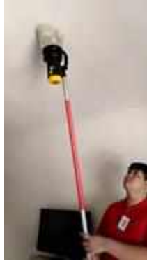
FL 11 ROOM 1119 TEST SMOKE DETECTOR 1 SET..NORMAL
