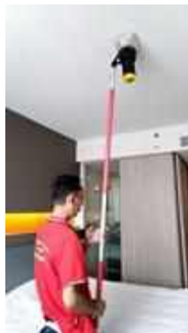
FL 23 ROOM 2319 TEST SMOKE DETECTOR 1 SET..NORMAL
