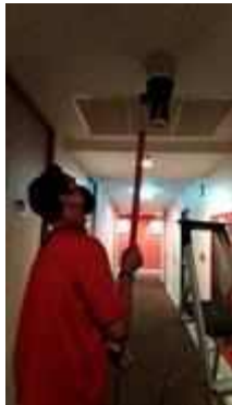
FL 19 CORRIDOR SERVICE TEST SMOKE DETECTOR 5 SET
