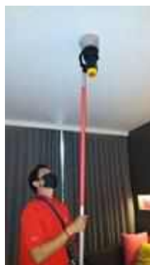
FL 26 ROOM 2619 SERVICE TEST SMOKE DETECTOR 1 SET
