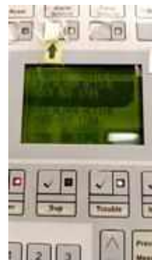
FL 28 ROOM 2805 TEST SMOKE DETECTOR 1 SET..NORMAL
