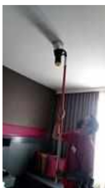
FL 27 ROOM 2710 SERVICE TEST SMOKE DETECTOR 1 SET
