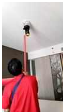
FL 25 ROOM 2519 SERVICE TEST SMOKE DETECTOR 1 SET
