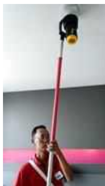
FL 24 ROOM 2418 TEST SMOKE DETECTOR 1 SET..NORMAL
