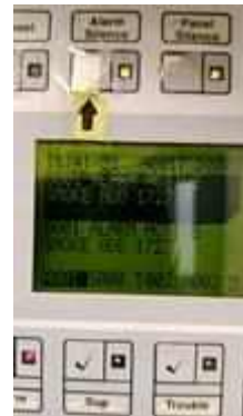
FL 17 ROOM 1714 TEST SMOKE DETECTOR 1 SET..NORMAL
