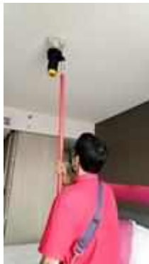
FL 27 ROOM 2712 SERVICE TEST SMOKE DETECTOR 1 SET
