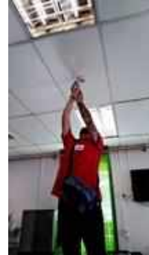
FL 8 CANTEEN SERVICE TEST SMOKE DETECTOR 2 SET NOWORK
