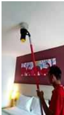
FL 17 ROOM 1714 TEST SMOKE DETECTOR 1 SET..NORMAL
