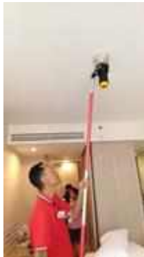
FL 25 ROOM 2502 TEST SMOKE DETECTOR 1 SET..
