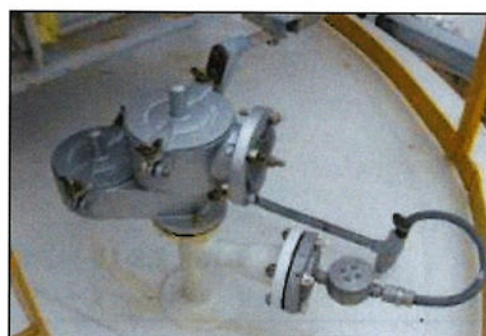
Pressure Vacuum Relief Valve
