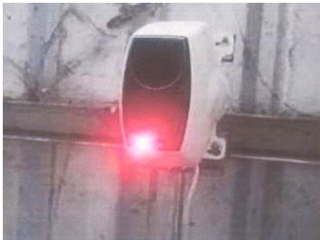
Smoke Beam Detector
