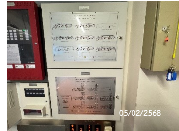
Graphic Annunciator Fire Alarm System
