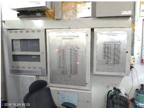
Fire Alarm Control Panel
