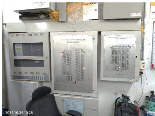
Fire Alarm Control Panel
