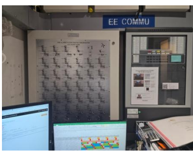
Graphic Annunciator Fire Alarm
