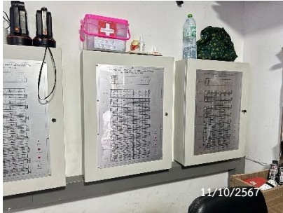
Graphic Annunciator Fire Alarm System
