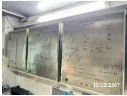
Graphic Annunciator Fire Alarm System
