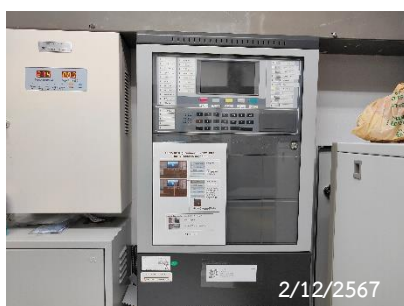
Fire Alarm Control Panel
