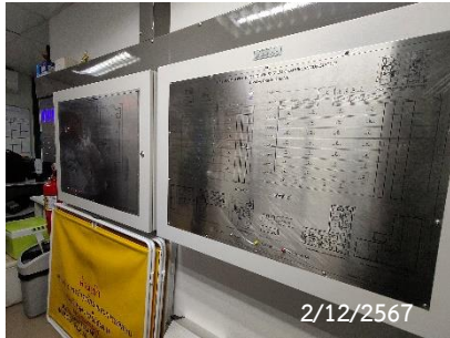
Graphic Annunciator Fire Alarm System
