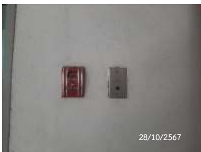
Fire Alarm Manual Station
