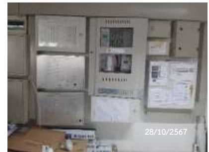
Graphic Annunciator Fire Alarm System
