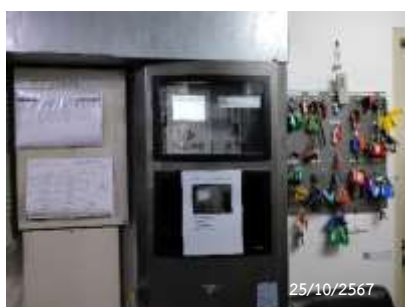
Fire Alarm Control Panel
