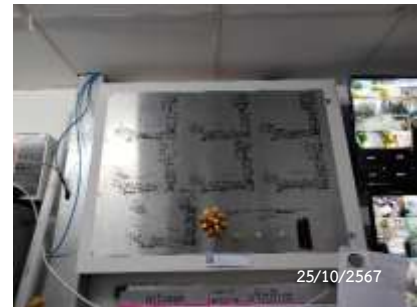
Graphic Annunciator Fire Alarm System
