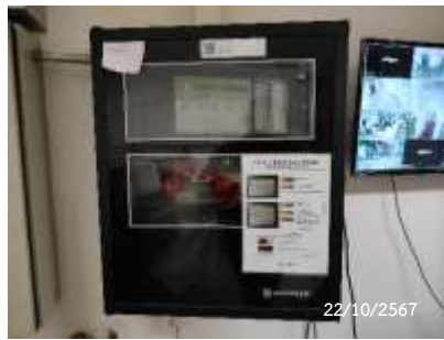
Fire Alarm Control Panel
