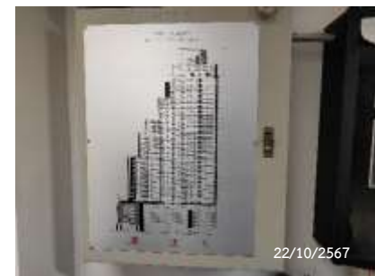
Graphic Annunciator Fire Alarm System
