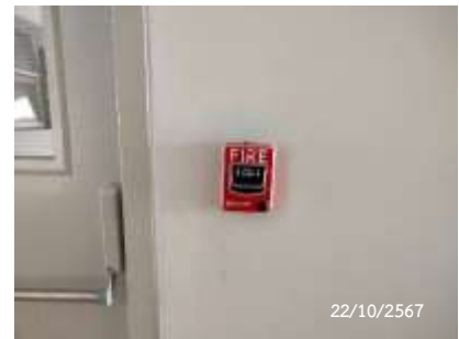
Fire Alarm Manual Station
