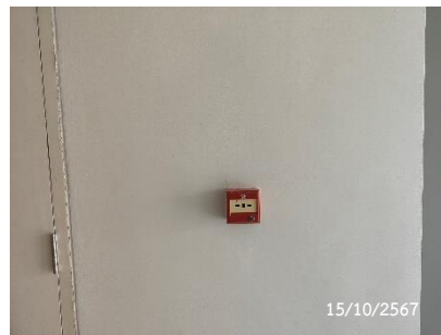
Fire Alarm Manual Call Point
