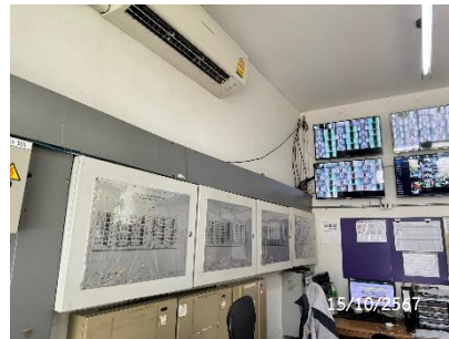
Graphic Annunciator Fire Alarm System
