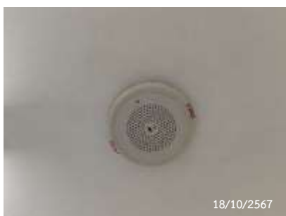
Fire Alarm Horn Strobe
