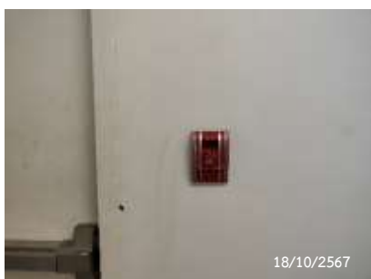
Fire Alarm Manual Station
