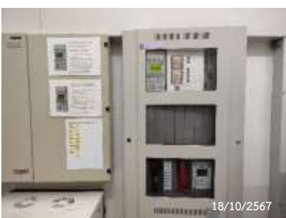
Fire Alarm Control Panel
