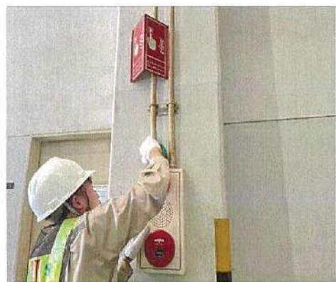
Combination Box (PLB) Cleaning
