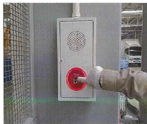
Combination Box (PLB) Testing and Decible
