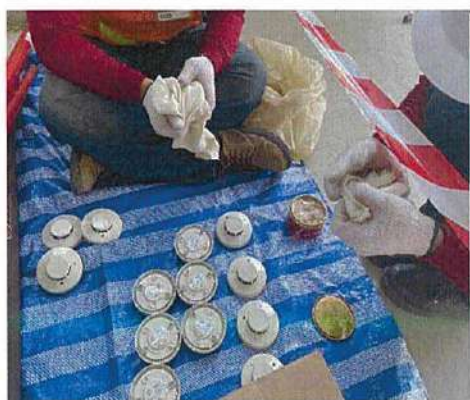
Smoke and Heat Detector Cleaning
