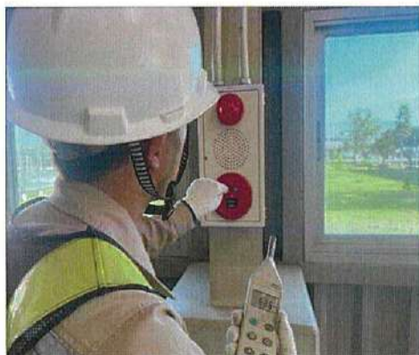
Combination Box (PLB) Testing and Decible
