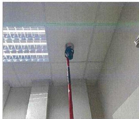
Heat Detector Testing
