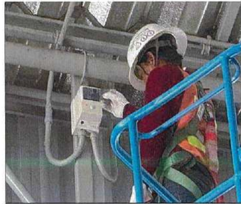
Smoke Beam Detector Testing
