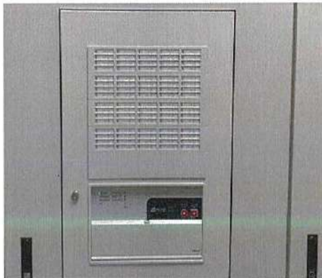
Fire Alarm Control Panel Normal
