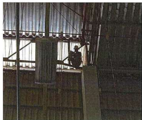
Smoke Beam Detector Cleaning
