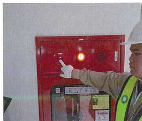
Combination Box (FHC) Testing and Decible
