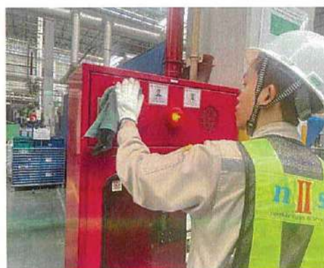
Combination Box (FHC) Cleaning
