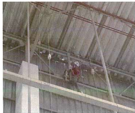
Smoke Beam Detector Testing
