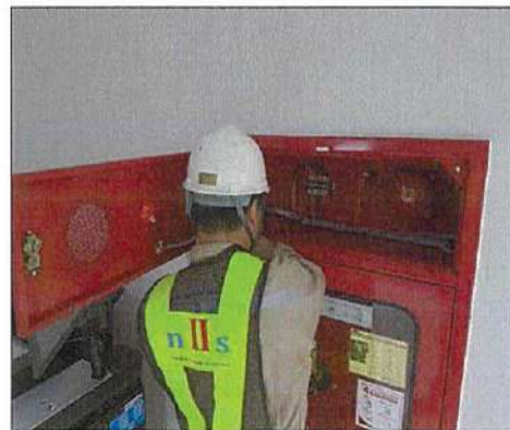
Combination Box (FHC) Cleaning
