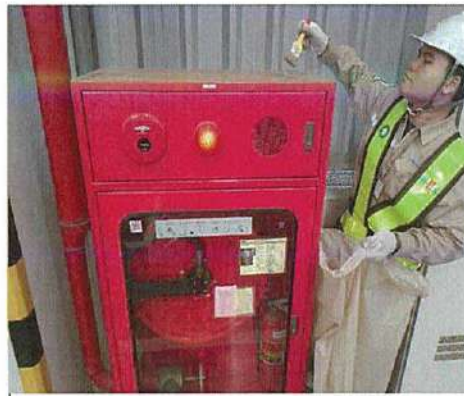
Combination Box (FHC) Cleaning
