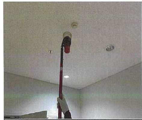
Smoke Detector Testing
