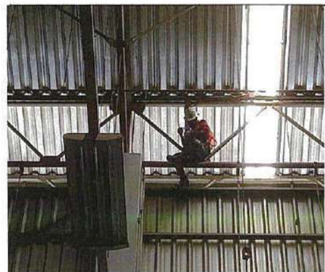
Smoke Beam Detector Cleaning
