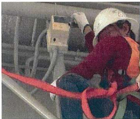
Smoke Beam Detector Testing
