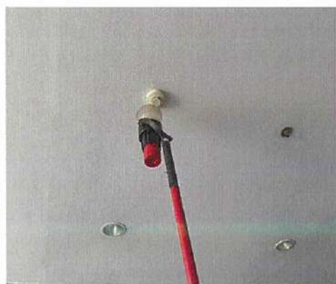
Smoke Detector Testing
