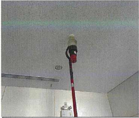
Smoke Detector Testing
