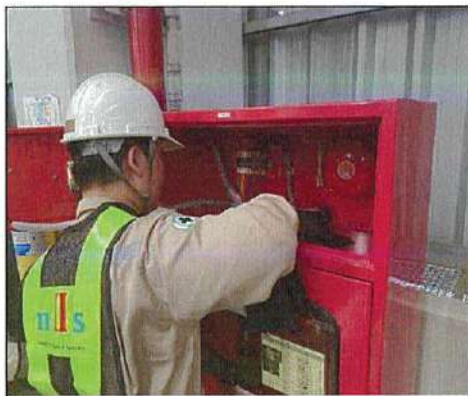
Combination Box (FHC) Cleaning
