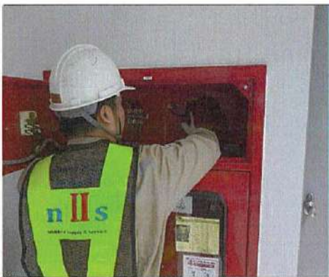
Combination Box (FHC) Cleaning
