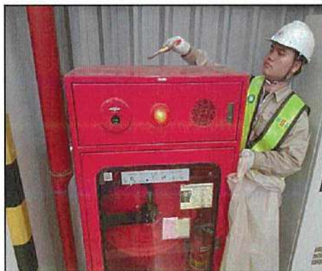
Combination Box (FHC) Cleaning
