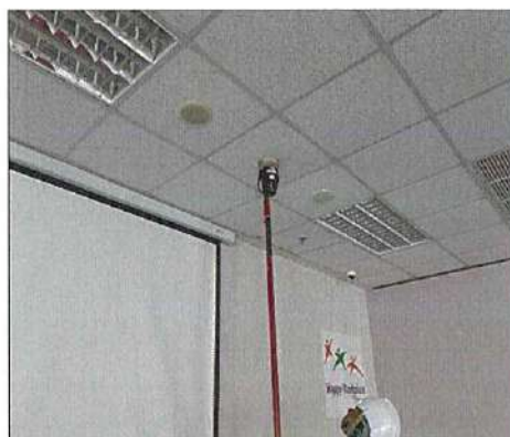
Heat Detector Testing
