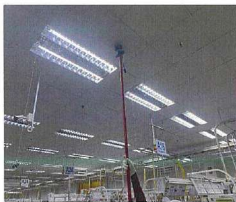
Remove Detector For Cleaning
