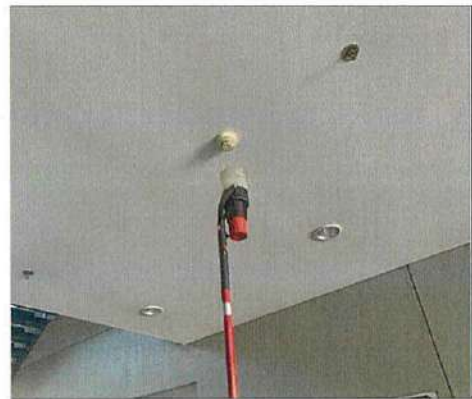
Smoke Detector Testing
