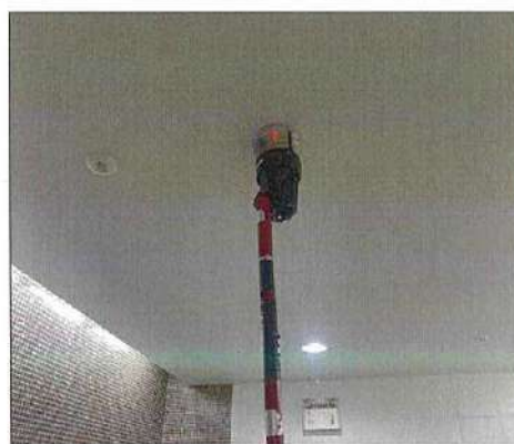
Heat Detector Testing
