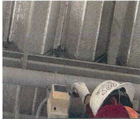
Smoke Beam Detector Testing
