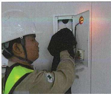
Combination Box (PLB) Cleaning
