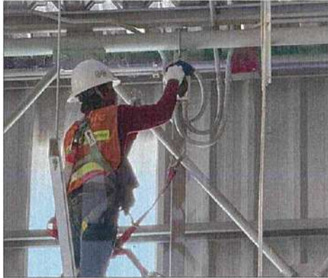
Smoke Beam Detector Cleaning
