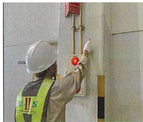
Combination Box (PLB) Cleaning
