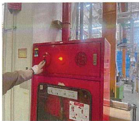
Combination Box (FHC) Testing and Decible
