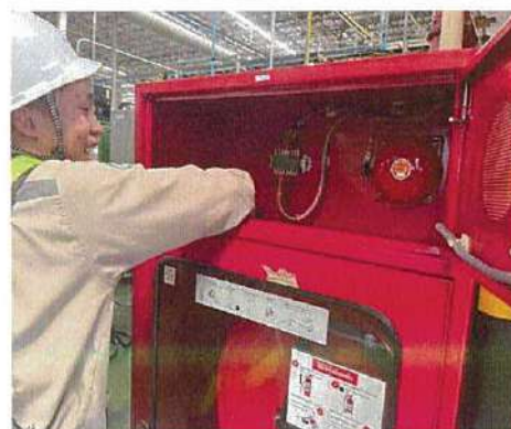
Combination Box (FHC) Cleaning
