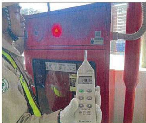
Combination Box (FHC) Testing and Decible
