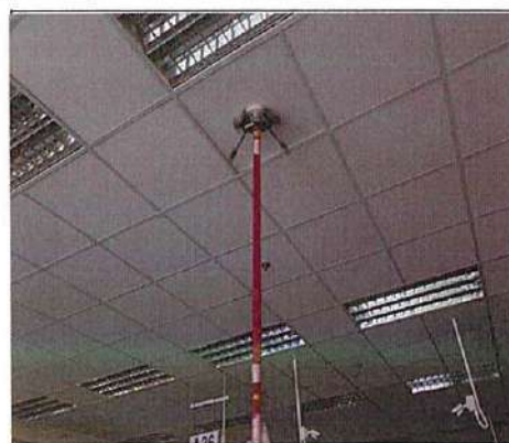
Remove Detector For Cleaning
