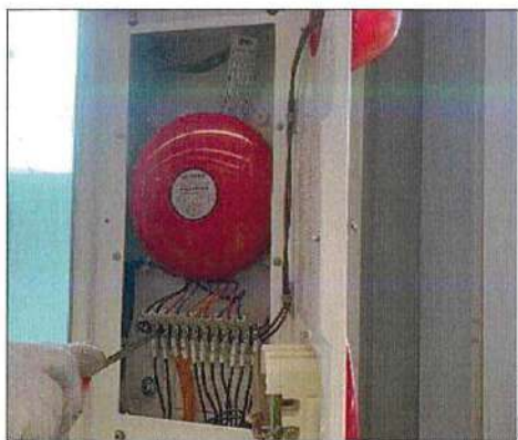
Combination Box (PLB) Checking
