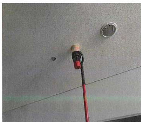
Smoke Detector Testing
