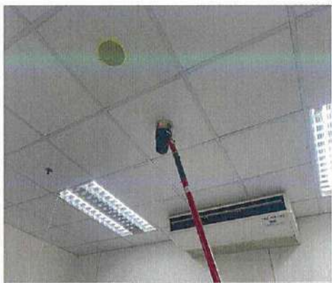
Heat Detector Testing
