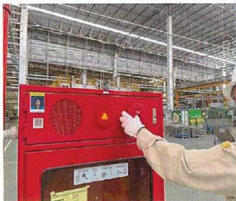
Combination Box (FHC) Testing and Decible
