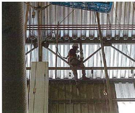
Smoke Beam Detector Cleaning
