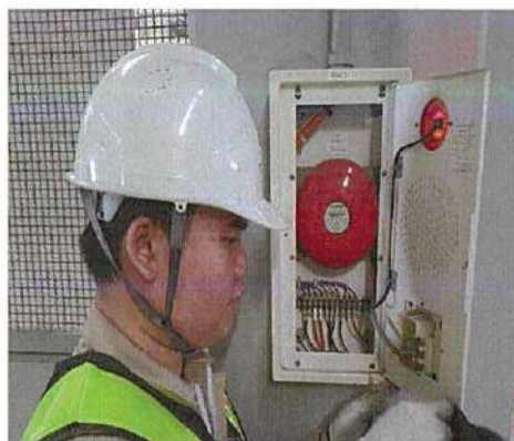
Combination Box (PLB) Checking
