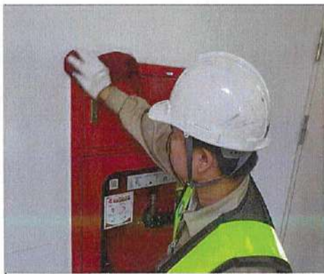
Combination Box (FHC) Cleaning
