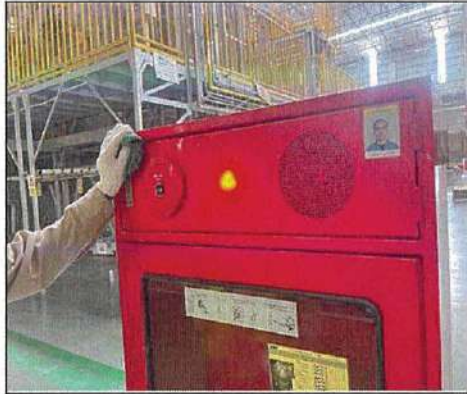
Combination Box (FHC) Cleaning
