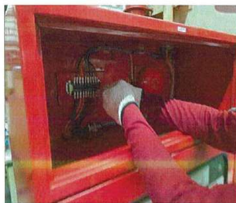
Combination Box (FHC) Checking
