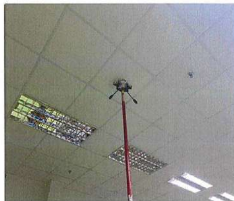
Remove Detector For Cleaning
