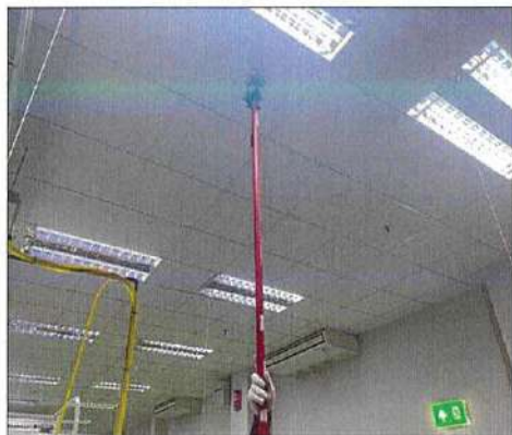
Remove Detector For Cleaning
