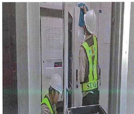
Fire Alarm Control Panel Cleaning
