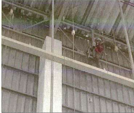
Smoke Beam Detector Cleaning
