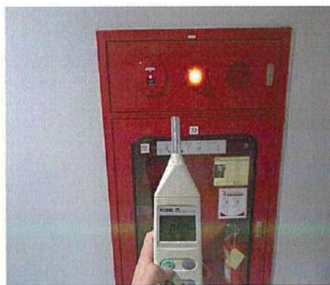
Combination Box (FHC) Testing and Decible
