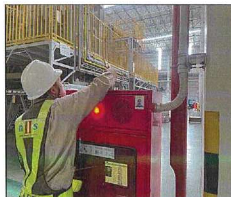
Combination Box (FHC) Cleaning
