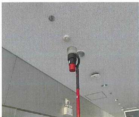
Smoke Detector Testing
