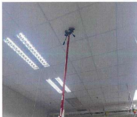
Remove Detector For Cleaning
