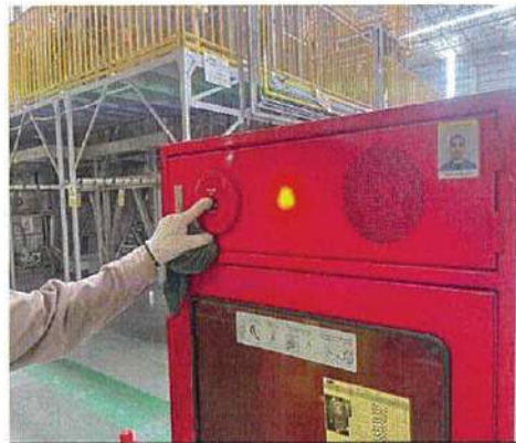
Combination Box (FHC) Testing and Decible
