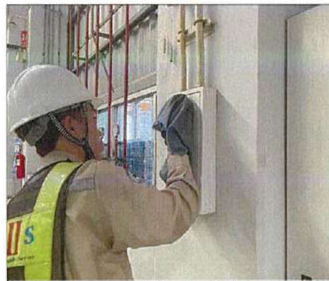
Combination Box (PLB) Cleaning
