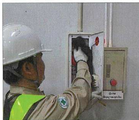
Combination Box (PLB) Cleaning
