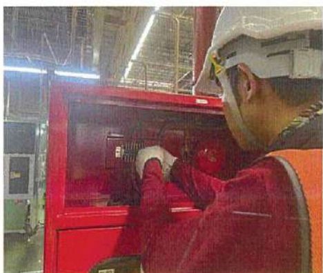
Combination Box (FHC) Checking
