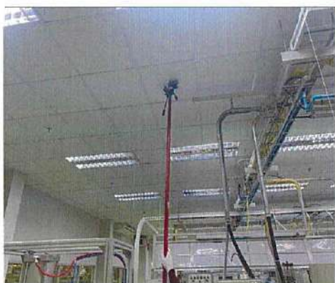
Remove Detector For Cleaning
