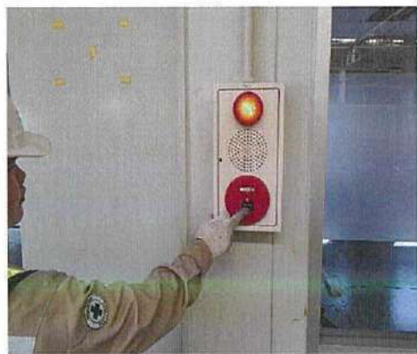
Combination Box (PLB) Testing and Decible
