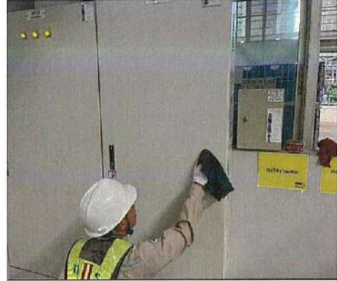
Terminal Box Cleaning
