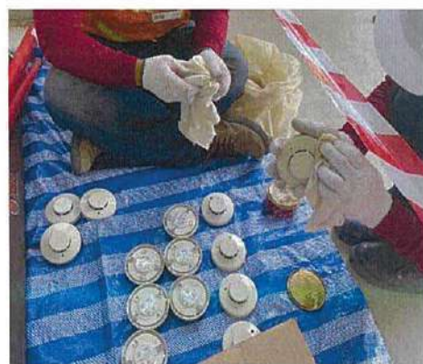
Smoke and Heat Detector Cleaning
