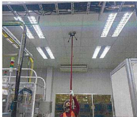
Remove Detector For Cleaning
