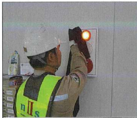
Combination Box (PLB) Cleaning
