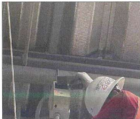
Smoke Beam Detector Testing
