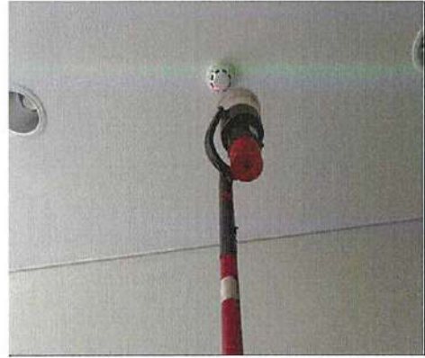
Smoke Detector Testing
