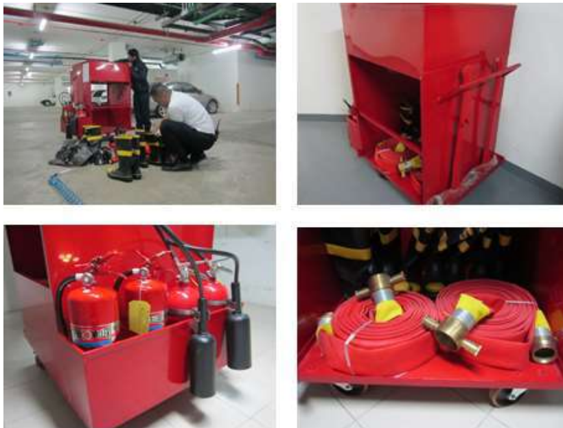
Portable Fire Extinguishers and Fire cart
