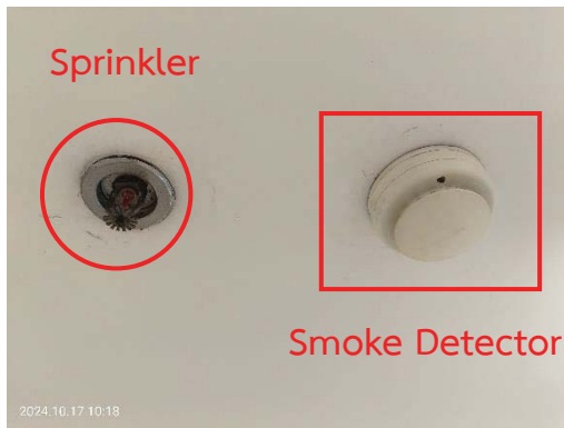
Smoke Detector & Sprinkler
