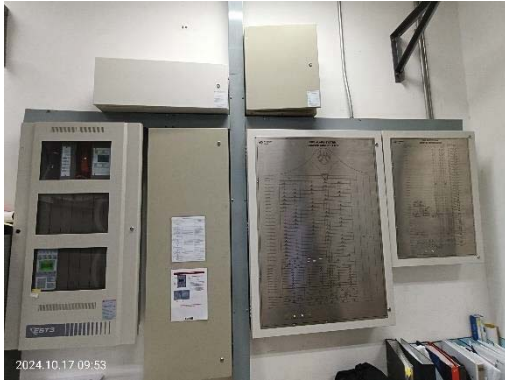
Fire Alarm Control Panel
