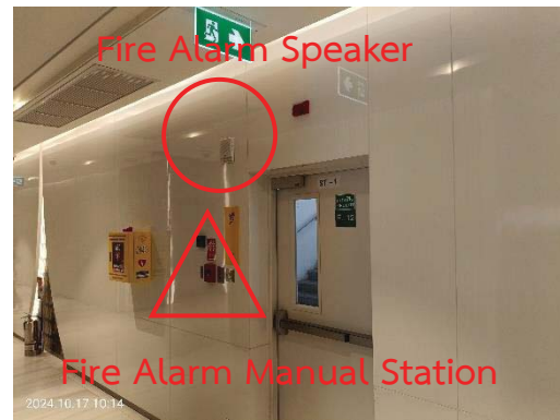
Fire Alarm Speaker & Fire Alarm Manual Station
