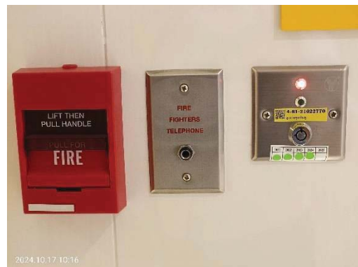
Fire Alarm Manual Station
