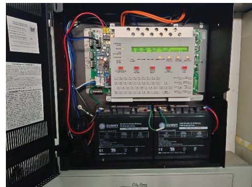
Fire Alarm Control Panel : FCP
