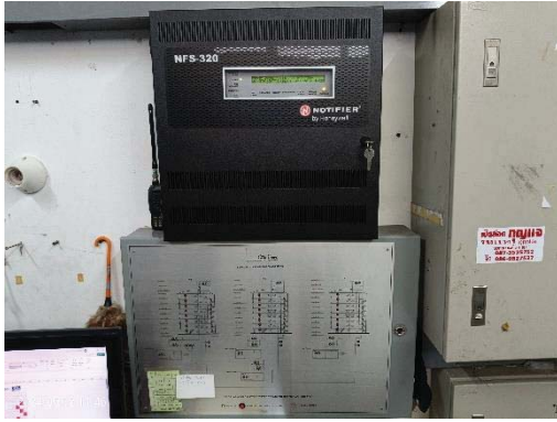
Fire Alarm Control Panel : FCP
