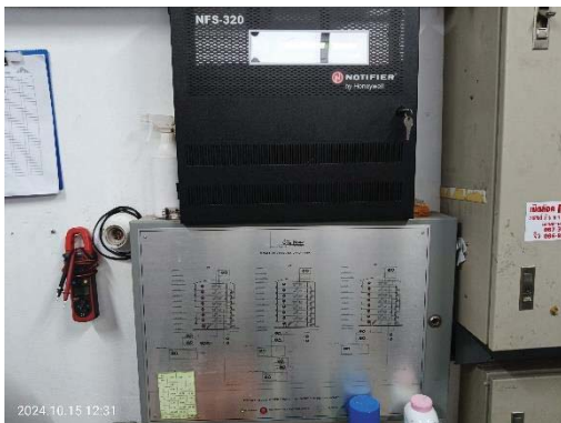
Fire Alarm Control Panel : FCP
