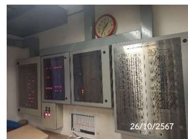
Graphic Annunciator Fire Alarm System
