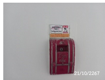
Fire Alarm Manual Station
