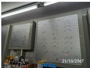
Graphic Annunciator Fire Alarm System
