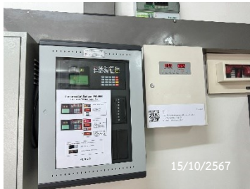
Fire Alarm Control Panel
