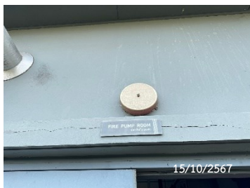
Sprinkler Fire Alarm When Bell Rings
