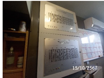
Graphic Annunciator Fire Alarm System
