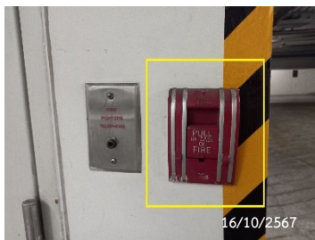
Fire Alarm Manual Station
