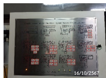
Graphic Annunciator Fire Alarm System
