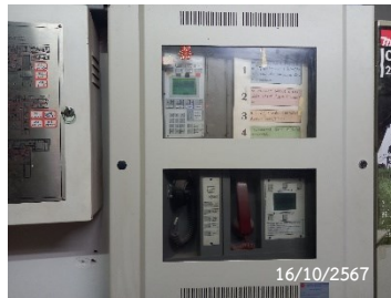
Fire Fighter Telephone System
