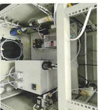
In CEMs cabinet there is so many dust and dirty and the filter in the cabinet's fan is so dusty
