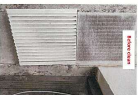
1.4 Image for fan filter in cabinet ( on the left of cabinet)
