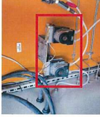
3. The Peristaltic pump ( we 're replaced the tube inside this pump )
