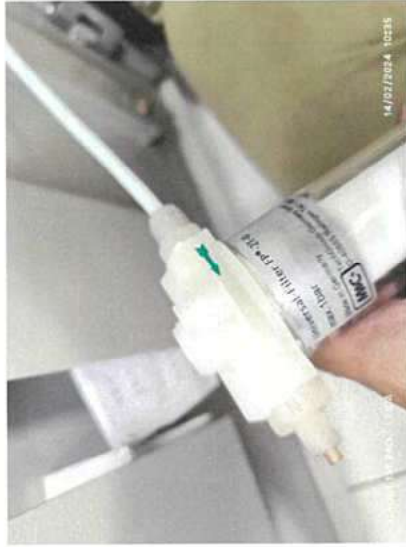
Model of moisture filter that replaced on boiler 1
