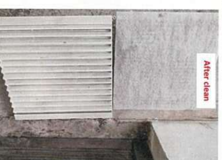
1.4 Image for fan filter in cabinet ( on the left of cabinet)
