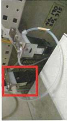
2. This solenoid valve is may have a problem when operate for switch to another port and temp. when operate is too high by the way this one could be a problem in the future ,for now it's fine to using it
