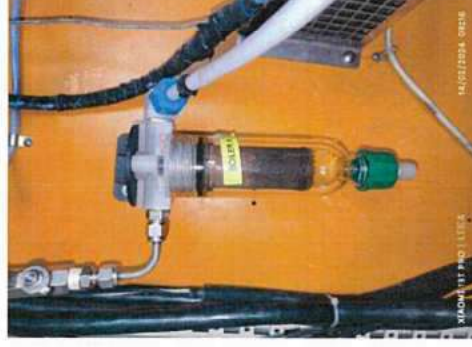
4. The moisture filter before and after replace
