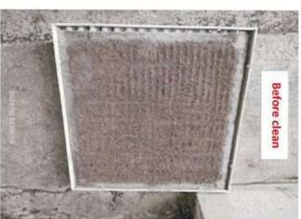
1.4 Image for fan filter in cabinet ( on the left of cabinet)
