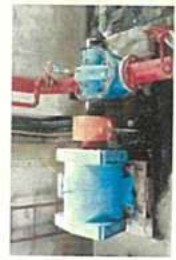
Motor Water Pumps, STP brand, Type TD12D 2969RPM, Head 102, Flow Meter 85 litres / Sec.
