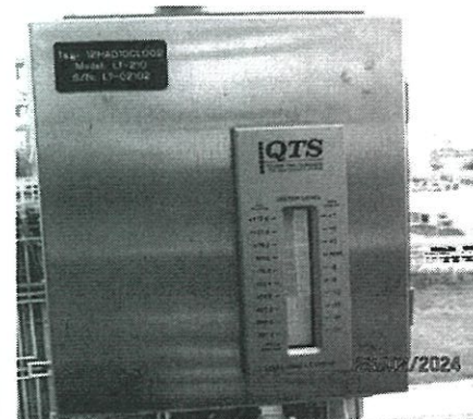
Water Level Indicator on Control Room
