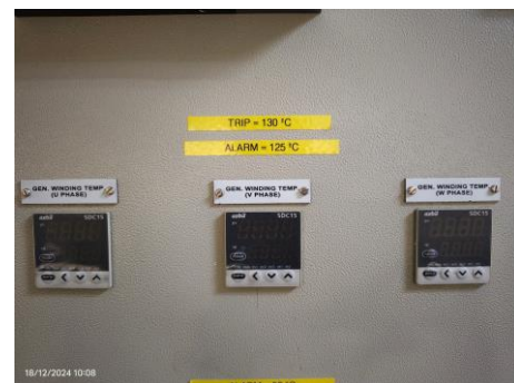
Temperature indicator for stator coils
