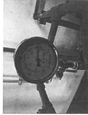
Figure 5.5 Fire pump running at 240 psi.
