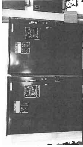
Figure 2.1 Control panel of fire pump.
